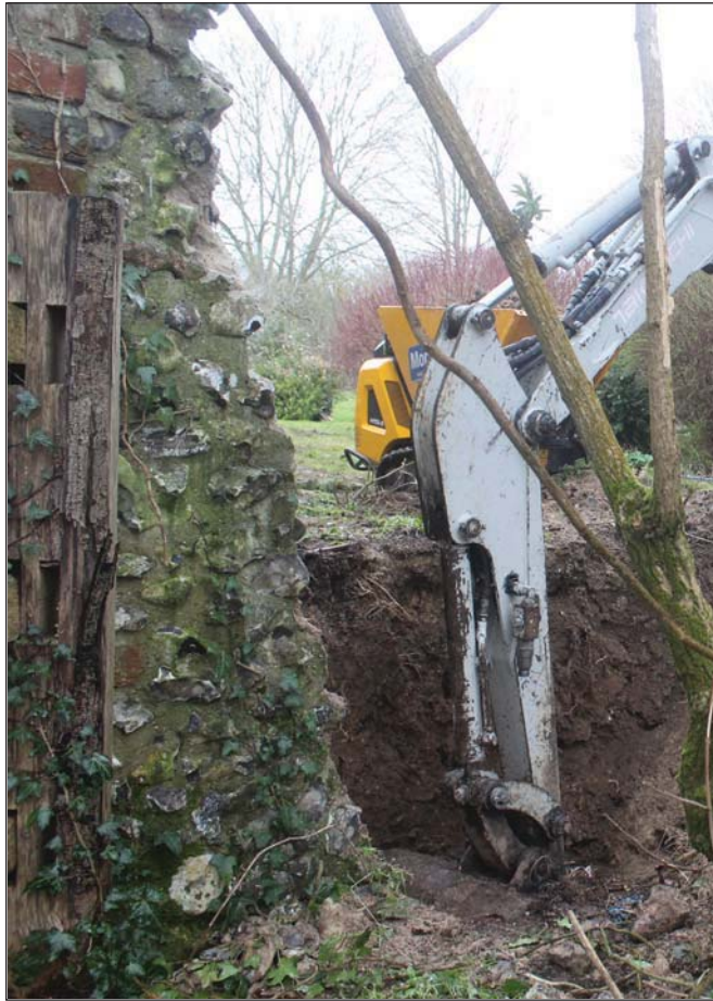
Plate 7. Removed wall shown abutting garden-room (left of photo), looking North-east.
