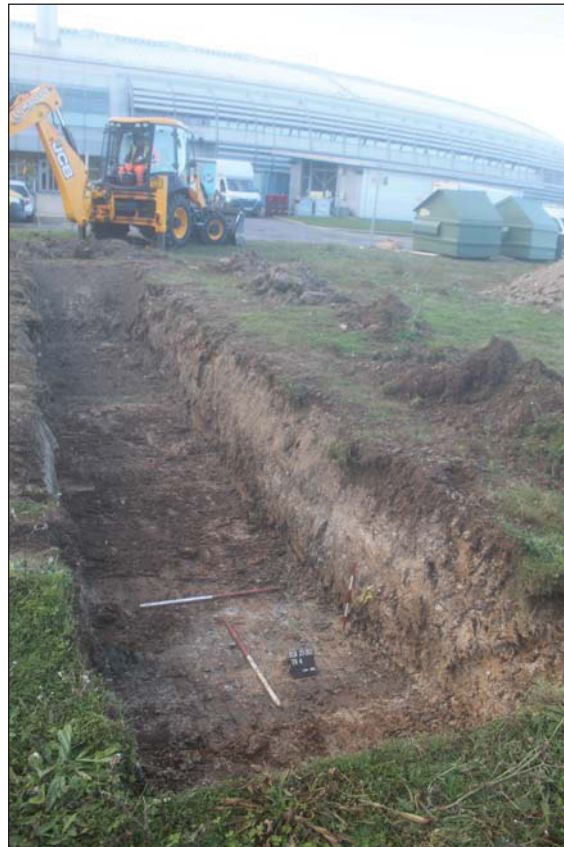
Plate 4. Trench 4, looking North West, Scales: 2x1m and 0.5m.
