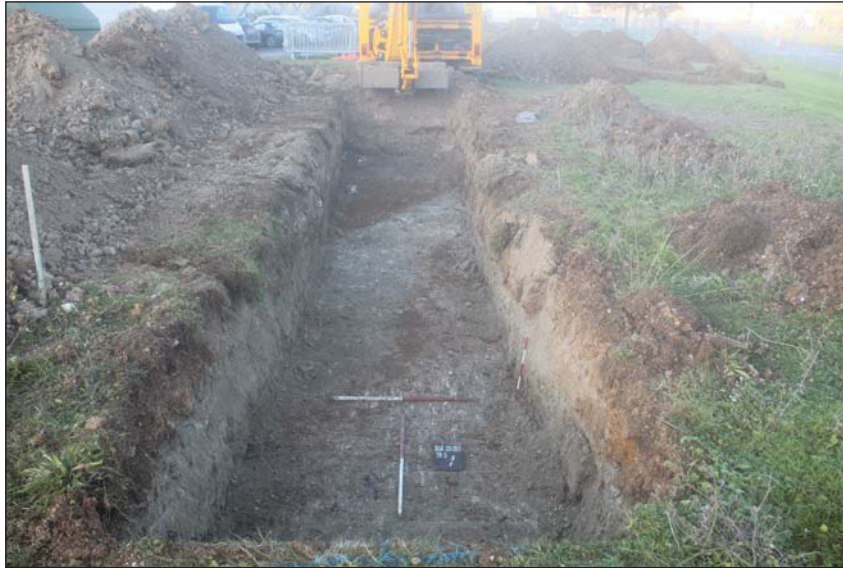
Plate 3. Trench 3, looking North West, Scales: 2x1m and 0.5m.
