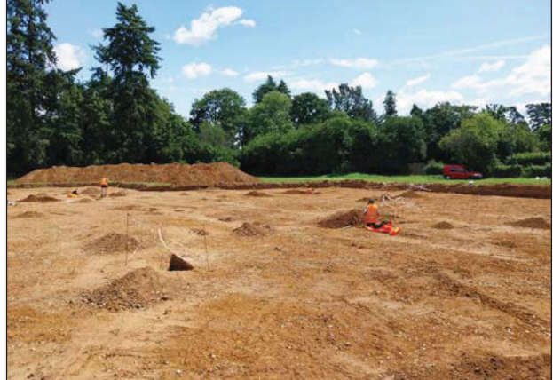
Plate 10. Working shot, looking south-east.
