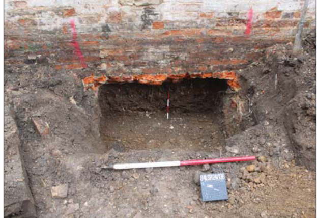
Plate 2. Underpinning Pit, looking East, Scales: 1m and 0.4m.
