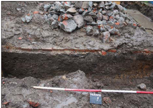
Plate 3. Foundation Trench, looking North, Scale: 2m.
