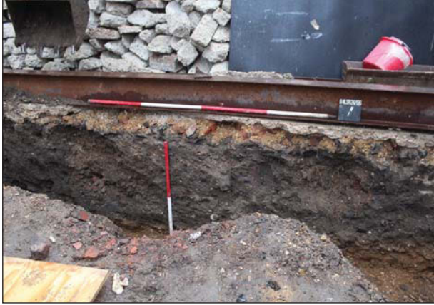
Plate 1. Foundation Trench, looking North, Scales: 2m and 1m.
