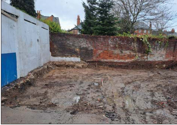
Plate 1. Ground reduction, looking west. Scales: 1m x2 and 0.4m
