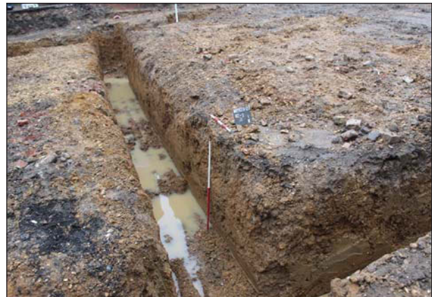
Plate 4. House 2/3 foundations, looking south-west. Scales: 1m and 0.5m..
