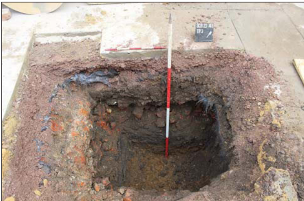
Plate 3. Test Pit 3, looking North-West, Scales: 2m and 0.5m.
