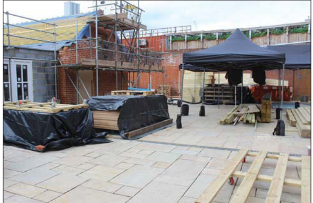
Plate 6. Site shot of already constructed extension and patio, looking North-West.
