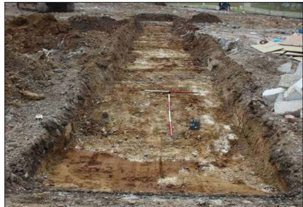
Plate 8. Trench 12, looking east south east. Scales: 2m, 1m and 0.3m.
