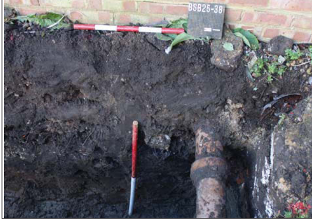
Plate 1. South-east side of foundation trench, looking east. Scales: 1m and 0.5m.
