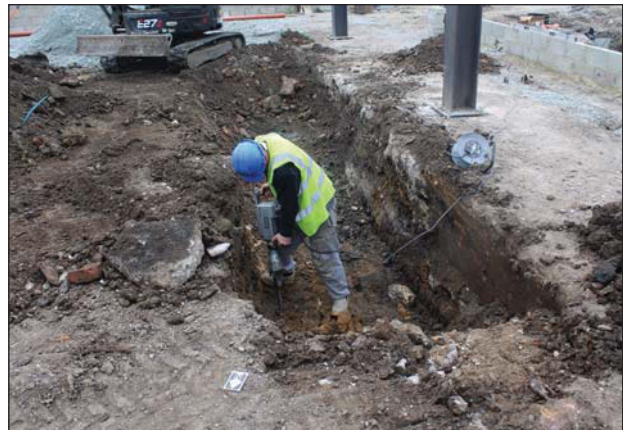
Plate 4. Trench excavation, looking southeast.
