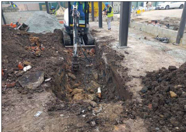
Plate 3. Trench excavation, looking southeast.
