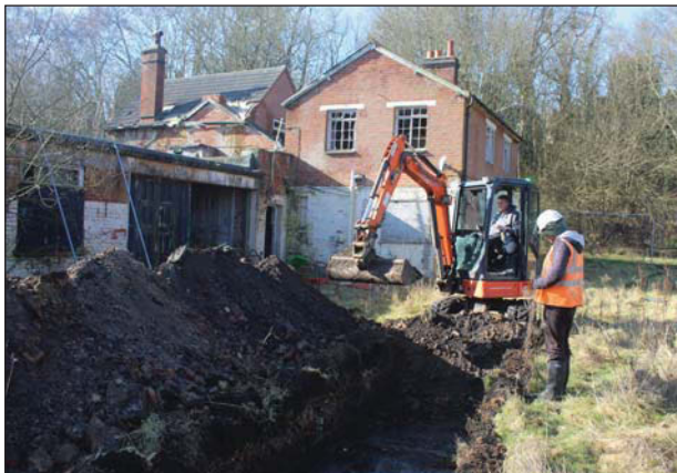
Plate 1. Working shot during excavation of Trench 1, looking West.
