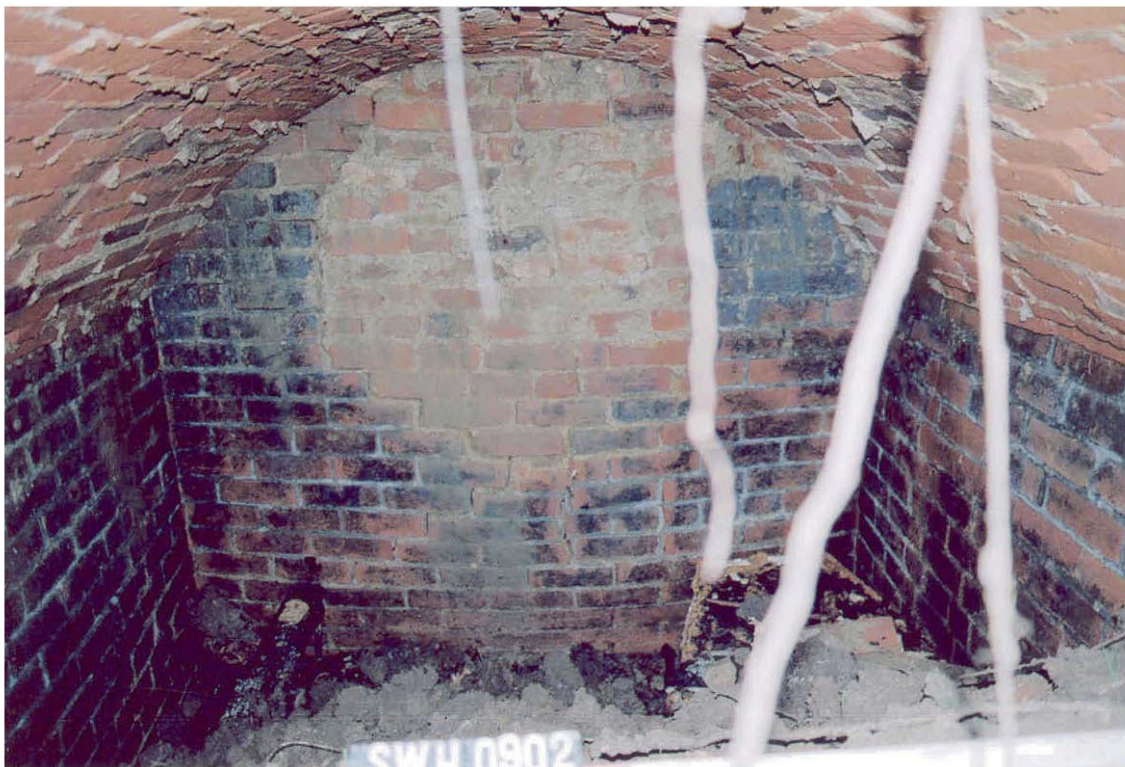
Plate 2. Crypt interior, showing wall repair and new vault.
