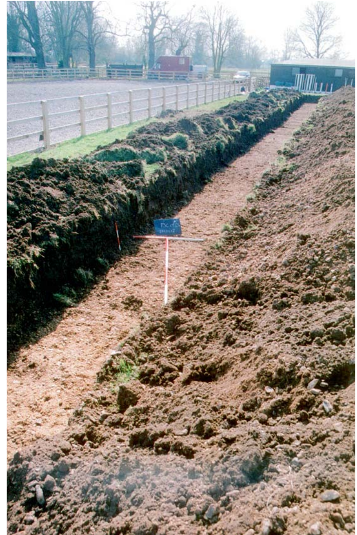
Plate 2. Trench 2, looking south, scales: 0.5m, 1m and 2m.
