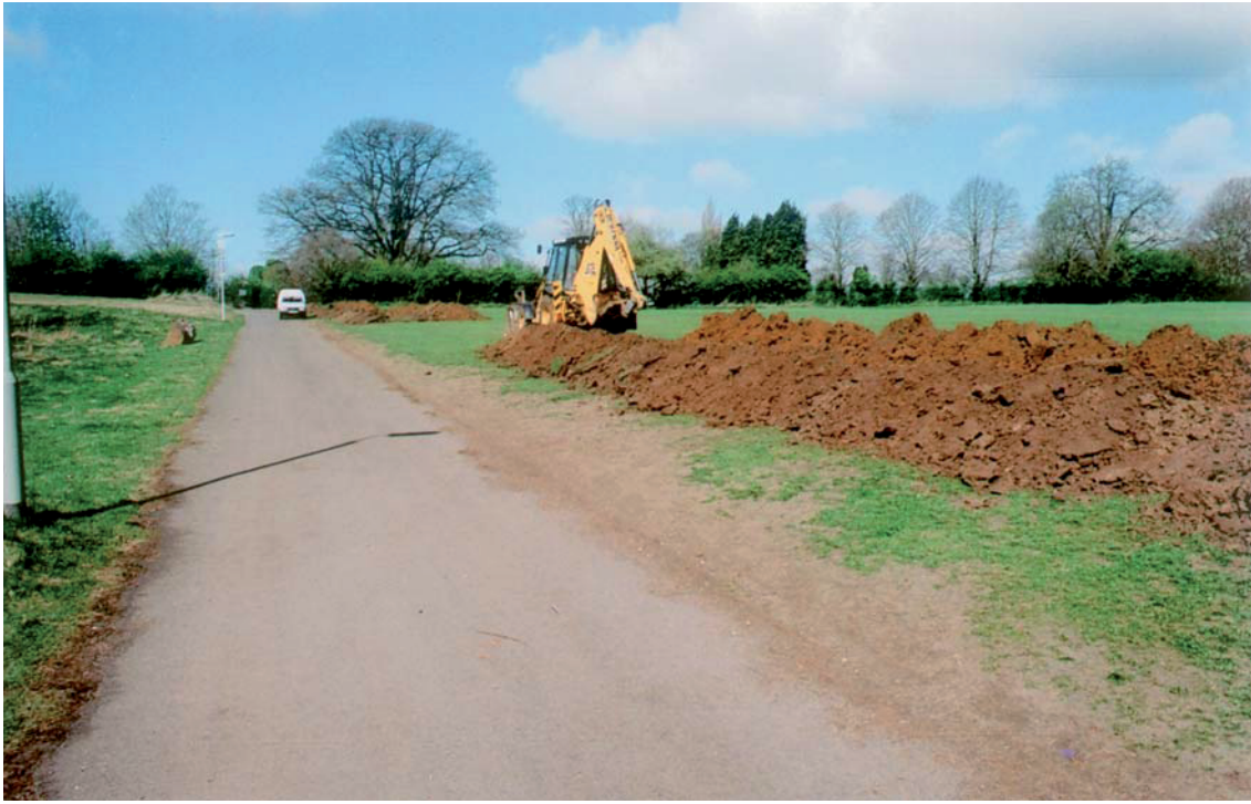
Plate 1. General site shot looking north west.
