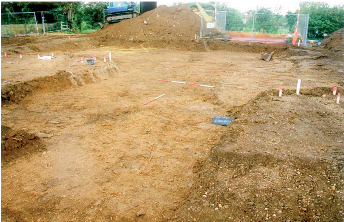
Plate 2. Road formation strip, looking west, scales: 2m and 1m.
