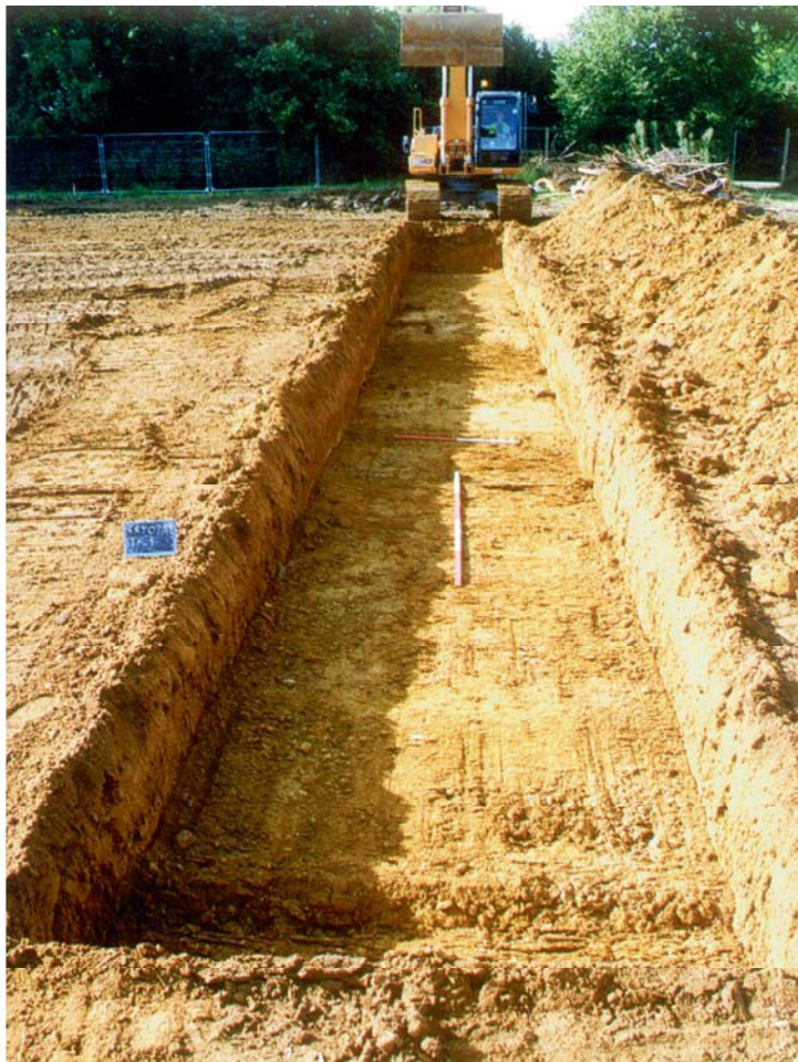
Plate 2. Trench 1, looking south, scales: 2m and 1m.
