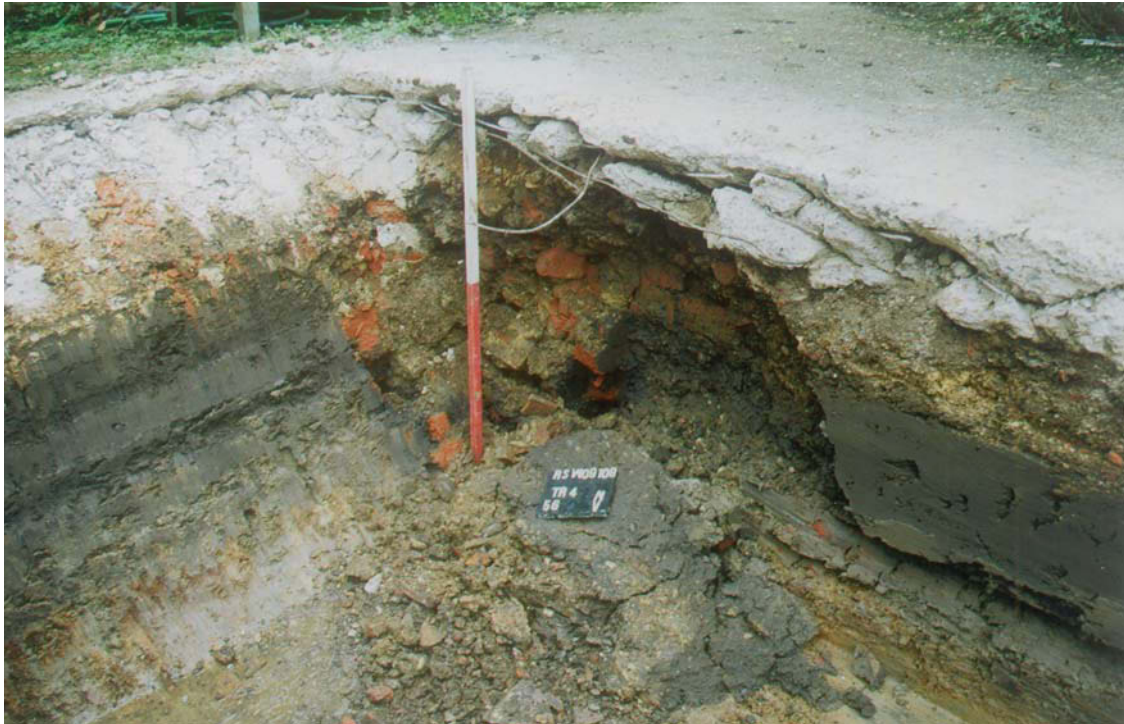
Plate 4. Trench 4, wall 56 in collapsed section, looking south-east, scale 1m.
