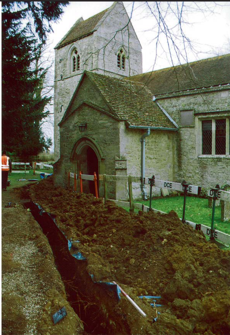
Plate 1. Sewer trench looking north-west, scale: 1m
