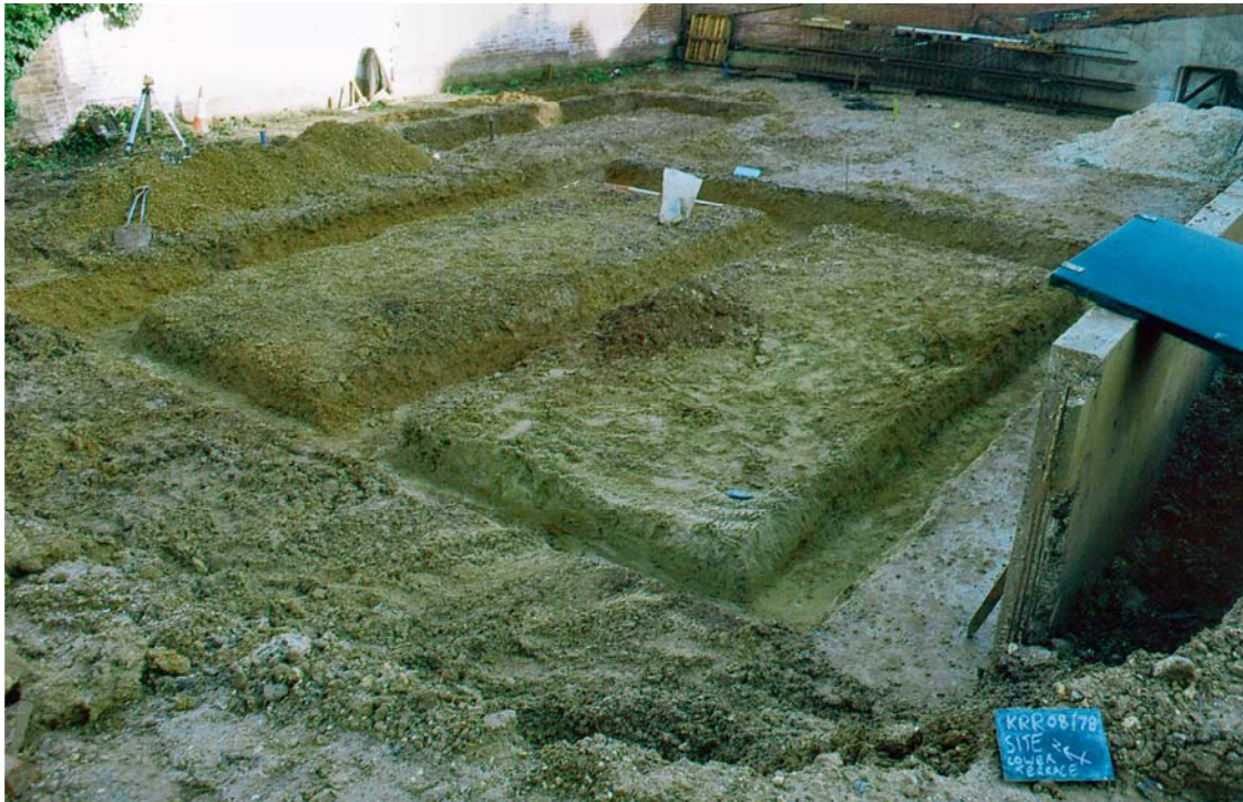
Plate 1. Plot 3 foundation trenches looking north east, scale: 2m
