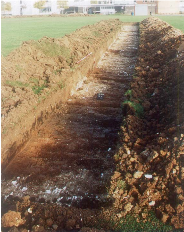
Plate 9. Trench 9, looking east north east, Scales 2m and 0.5m.
