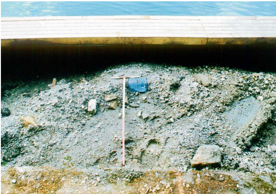
Plate 2. Dredged material placed behind piling, looking west, scales 0.3m, 1.0m
