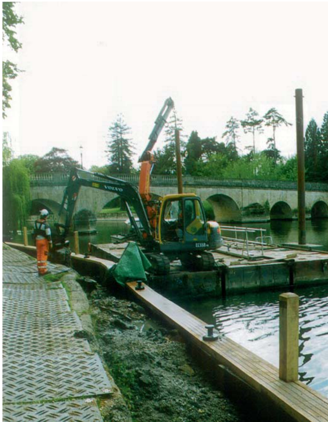
Plate 1. General view, looking south towards Wallingford Bridge, showing dredging in progress.
