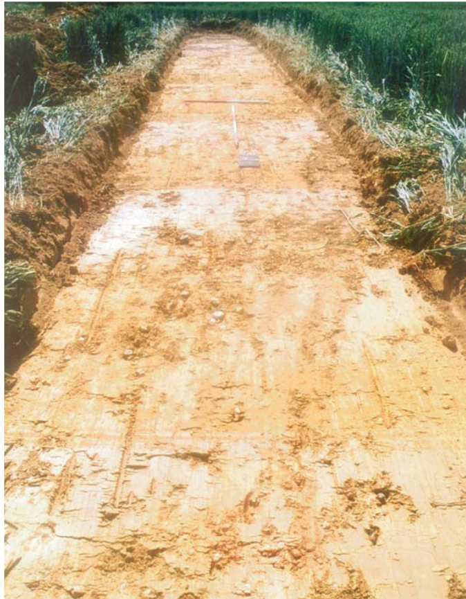
Plate 4. Trench 60, looking south-west. scales: horizontal 2m and 1m, vertical 0.3.
