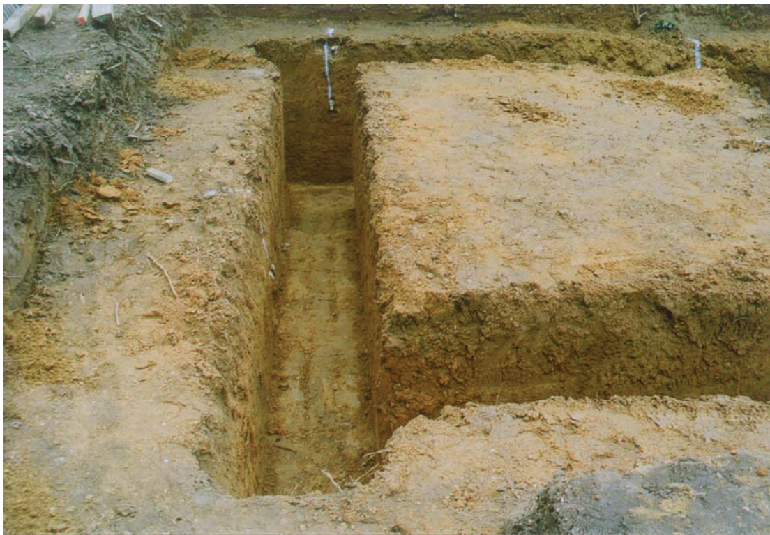
Plate 2. Plot 1, typical area of footing trench, looking west.
