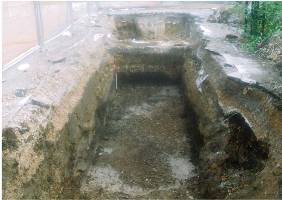
Plate 1. Trench 1, looking north east, scales; horizontal 1m, vertical 1m.
