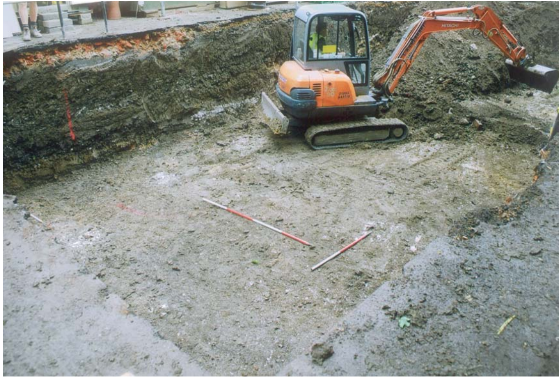
Plate 1. Soakway excavation, looking north-west, scales: 1m and 2m.
