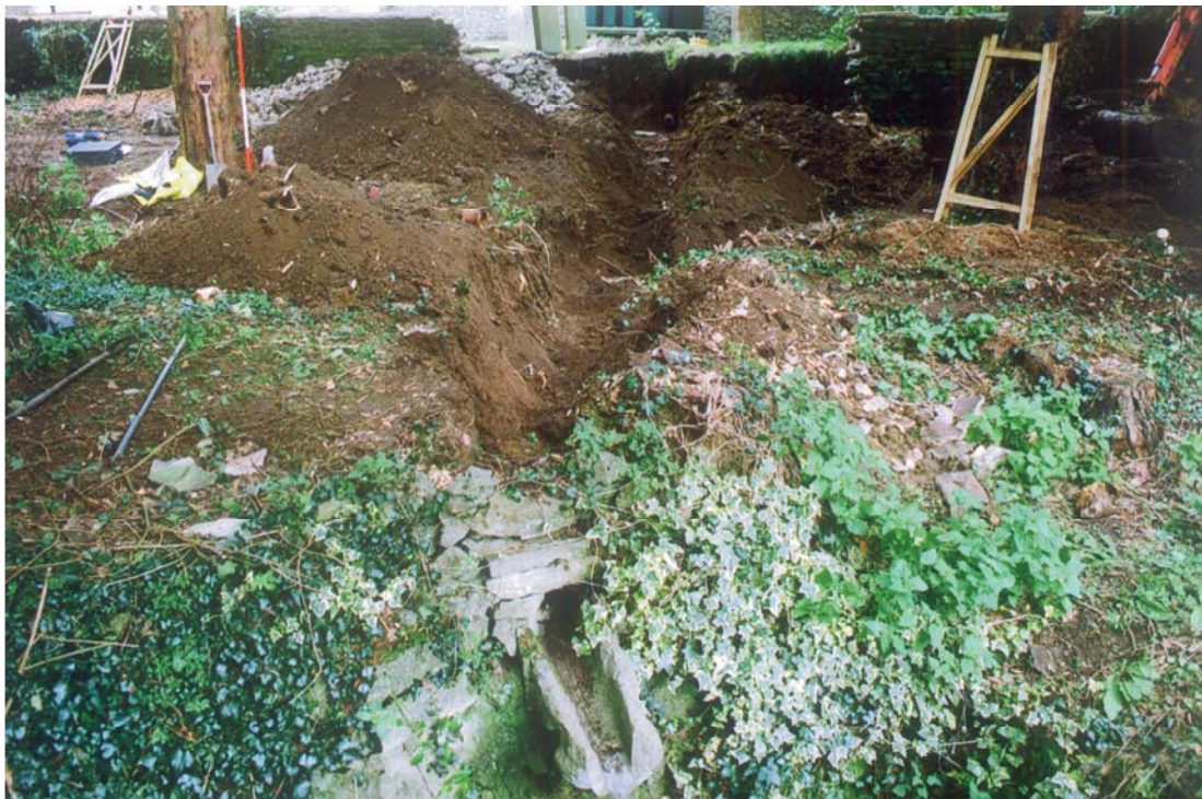
Plate 4. Surface water outflow pipe, showing line of removed pipe.
