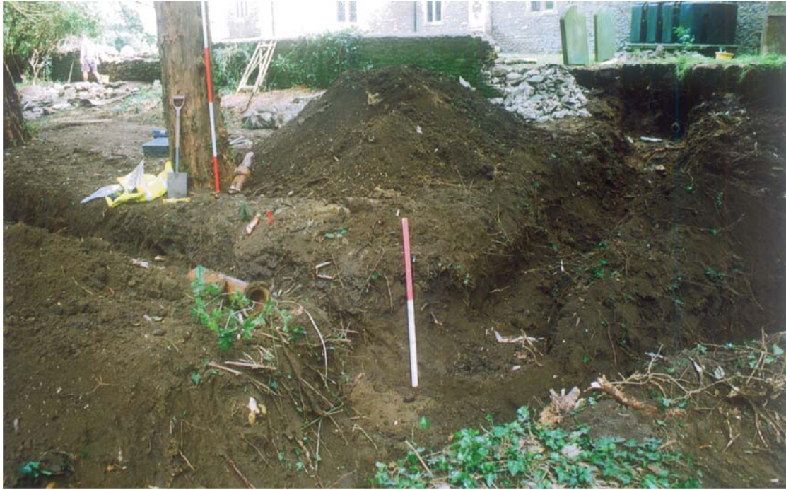
Plate 3. Surface waterpipe trench crossing boundary wall trench, looking east; scale 1m.
