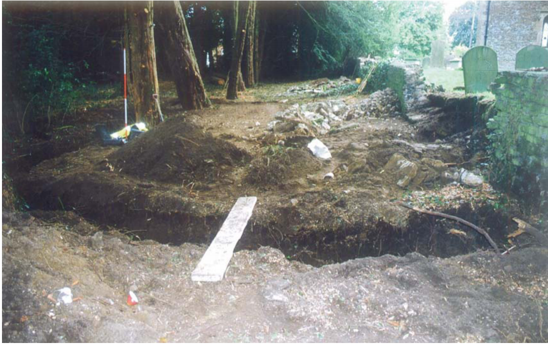
Plate 1. Works, looking north east.
