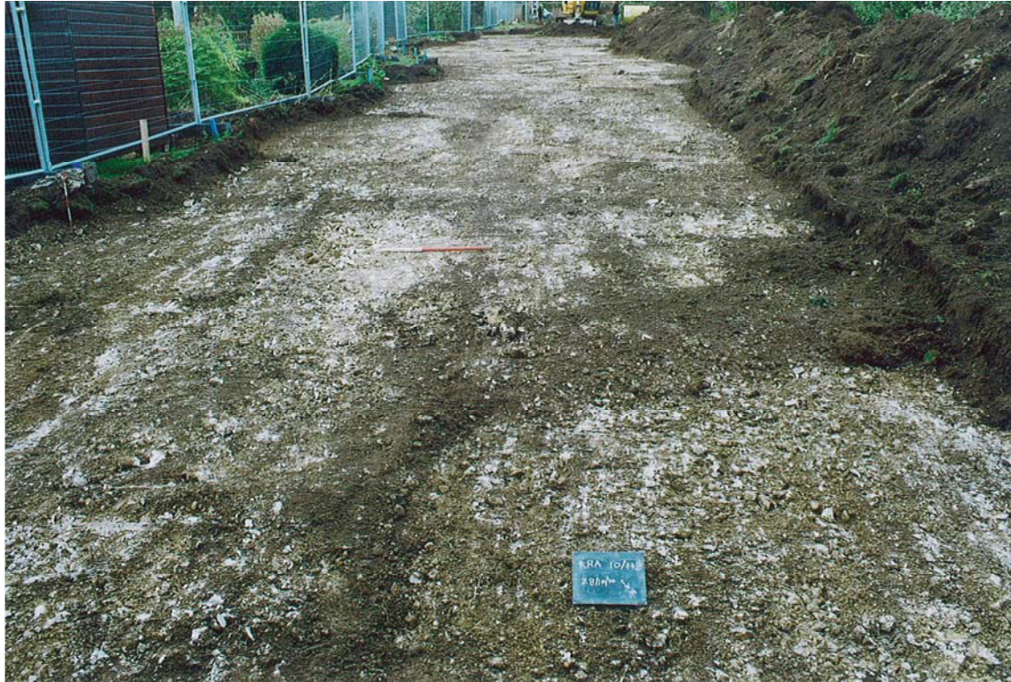
Plate 1. Stipping of initial road corridor of site adjacent to south eastern boundary, looking south west.
