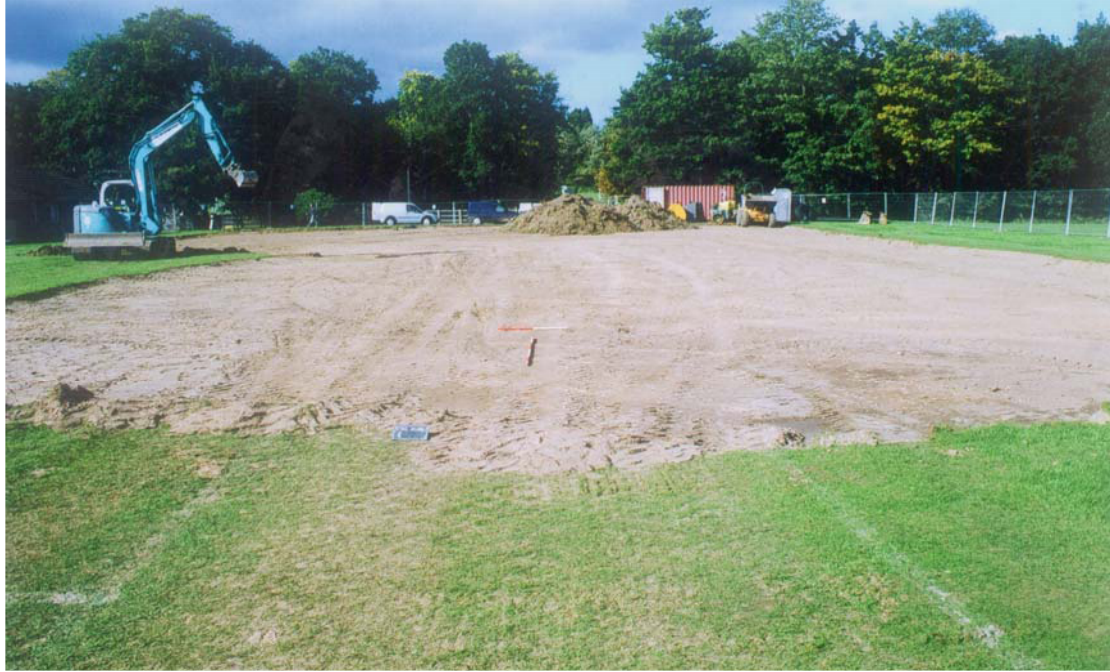
Plate 1. General view of area strip looking north.
