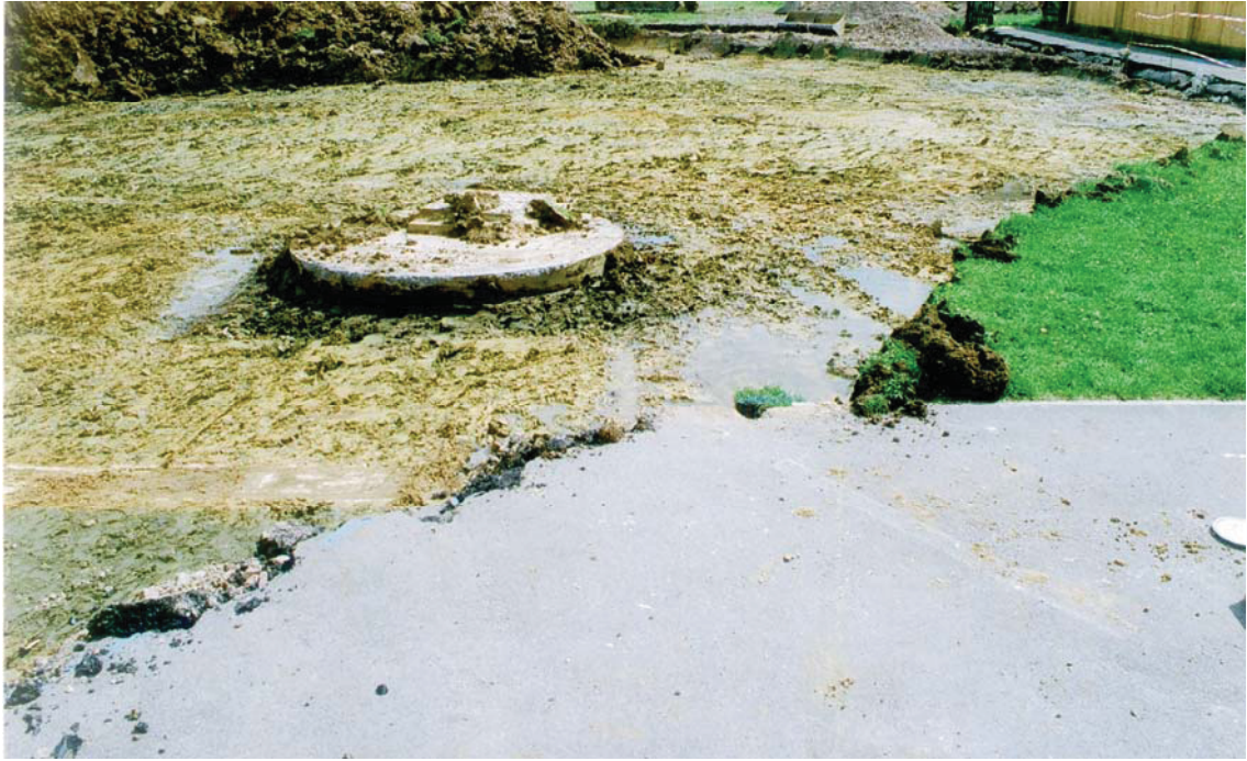
Plate 1. Drain in stripped area, looking south.
