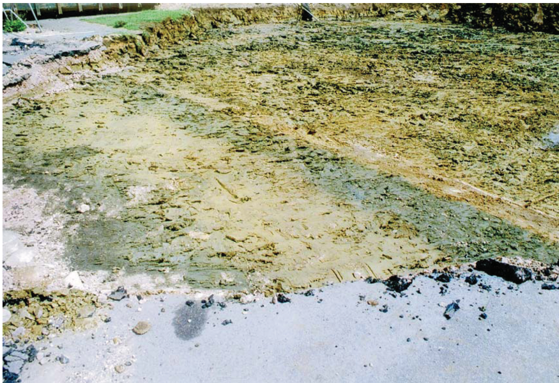
Plate 2. Linear disturbance, looking south south east.
