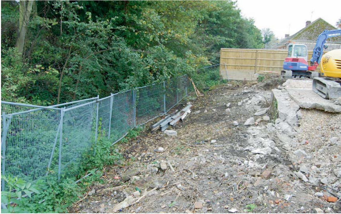
Plate 1. General view down existing earthwork ditch, looking south
