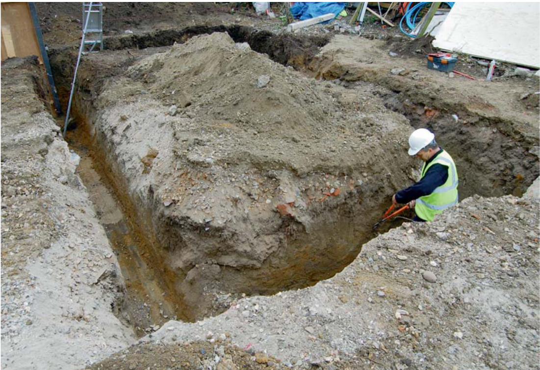
Plate 2. Footing trenches for southern plot, looking south east.
