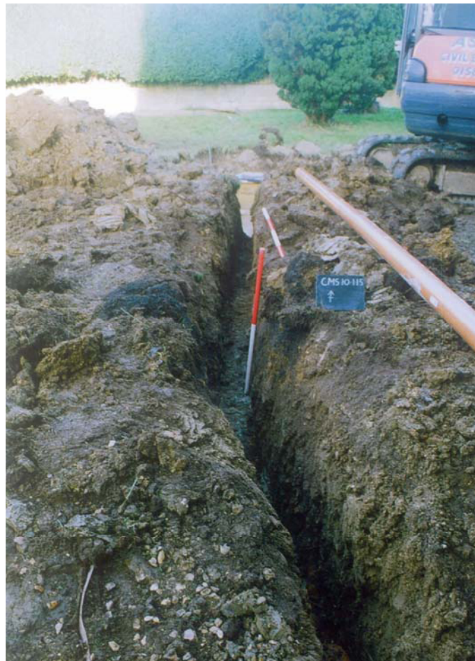
Plate 4. Service Trench, looking north, Scales: 1.0m and 1.0m
