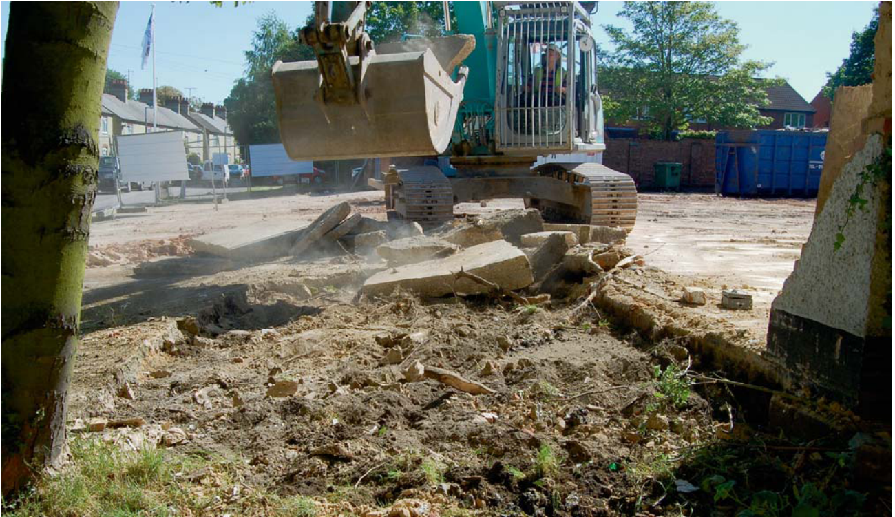
Plate 1. Former yard, looking south east
