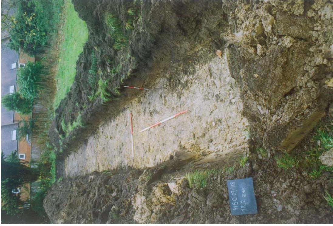
Plate 1. Trench 2, looking east, scales: 2m, 1m and 0.5m.
