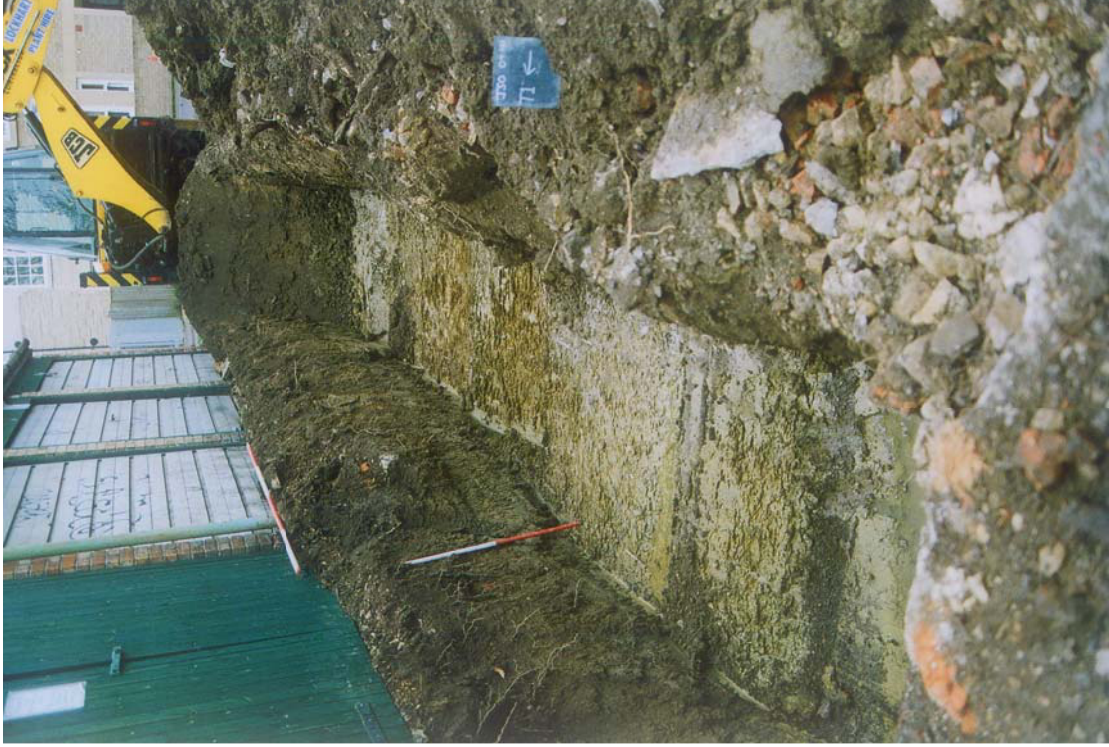
Plate 1. Trench 1, looking east, scales: 1m and 2m.
