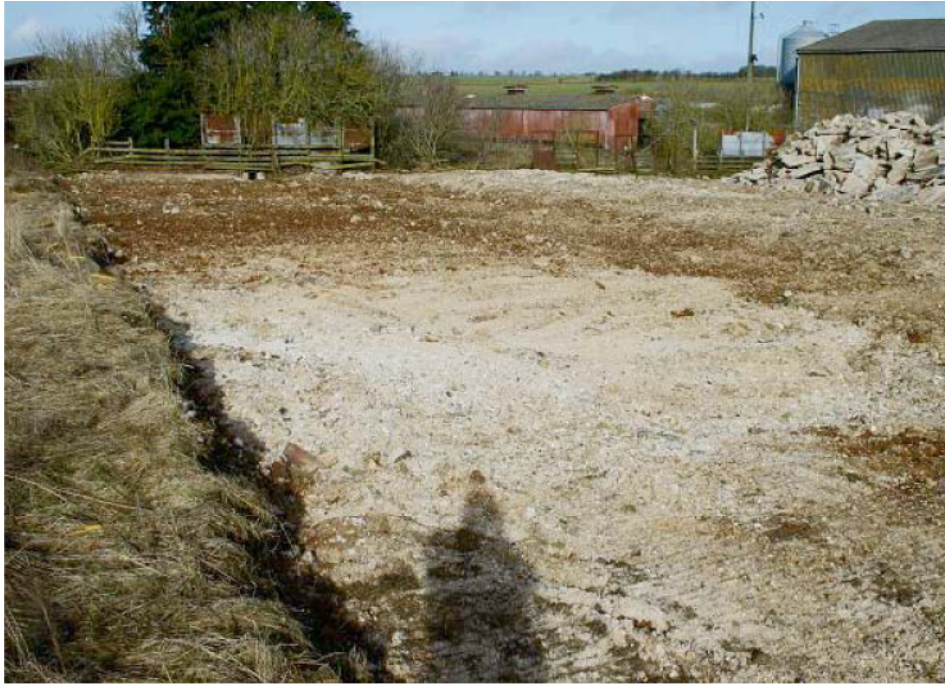
Plate 1. Levelled area of barn, looking north.
