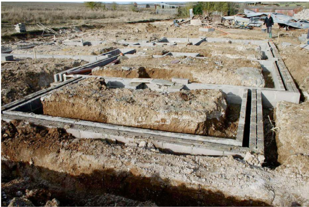
Plate 2. General view over top of house footings, looking north.
