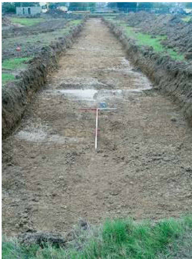
Plate 1. NE Road strip, looking south west. Scales 2m and 1m.
