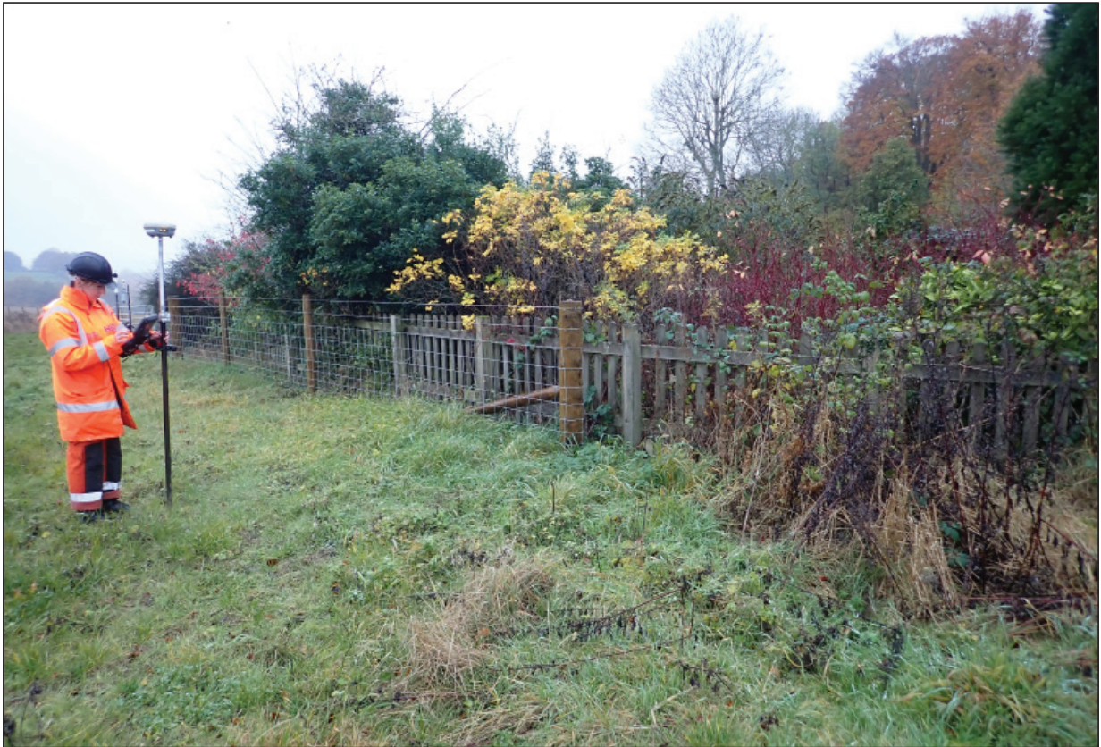
Plate 1 - Working shot looking south, showing newly installed fence on the eastern side of the Site
