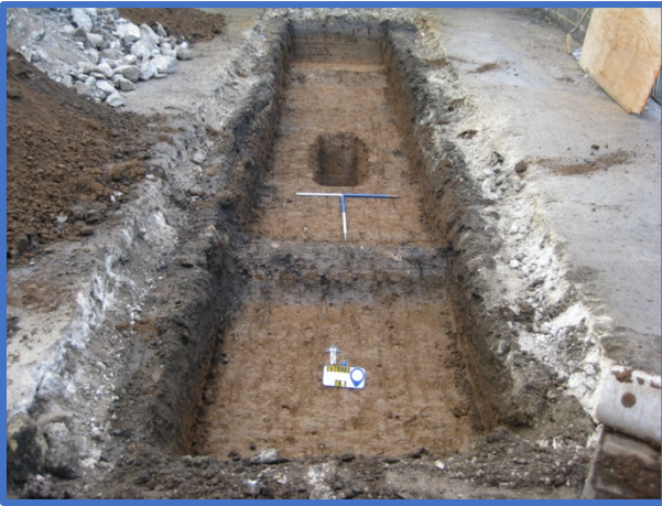
Plate 2. Trench 1, blank with services and test pit, looking E, w
