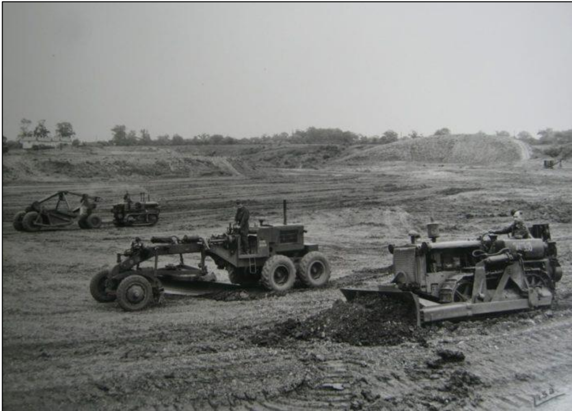
Plate 8 Airfield construction in Hertfordshire - 1941, showing the levelling of the land.
