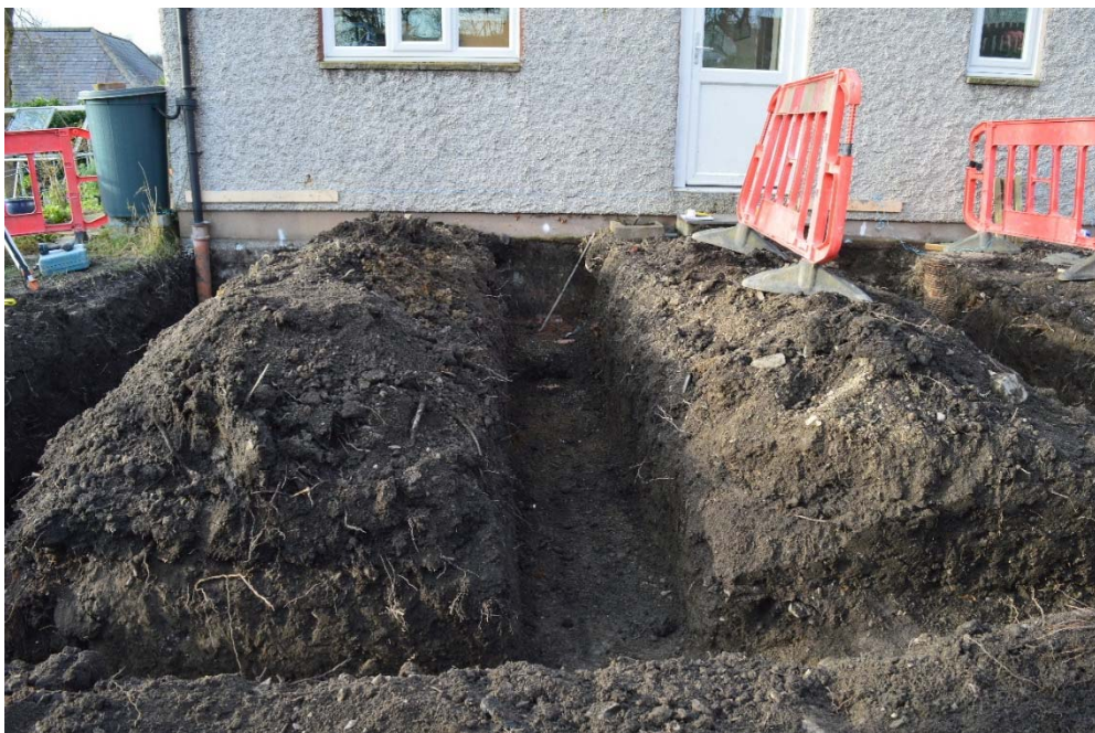
Fig. 4. View from the east of groundworks following completion CPAT 4121-0005.
