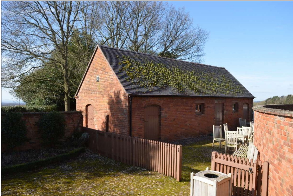
Fig. 3 The 19th century farm building (now a cafeteria) to the south-west of the farmyard. Photo CPAT 4482-0007
