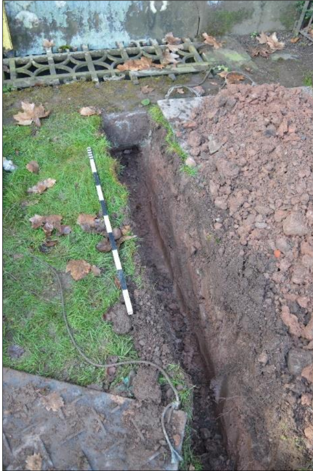
Fig. 4 cable trench and light well for Gatehouse cellar
