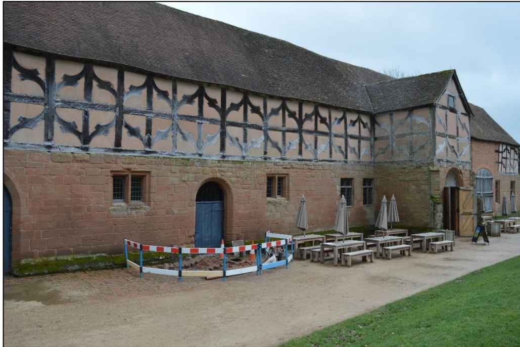
Fig. 2 View of the stables from the north-east, showing the location of the groundworks. Photo CPAT 4607-0006
