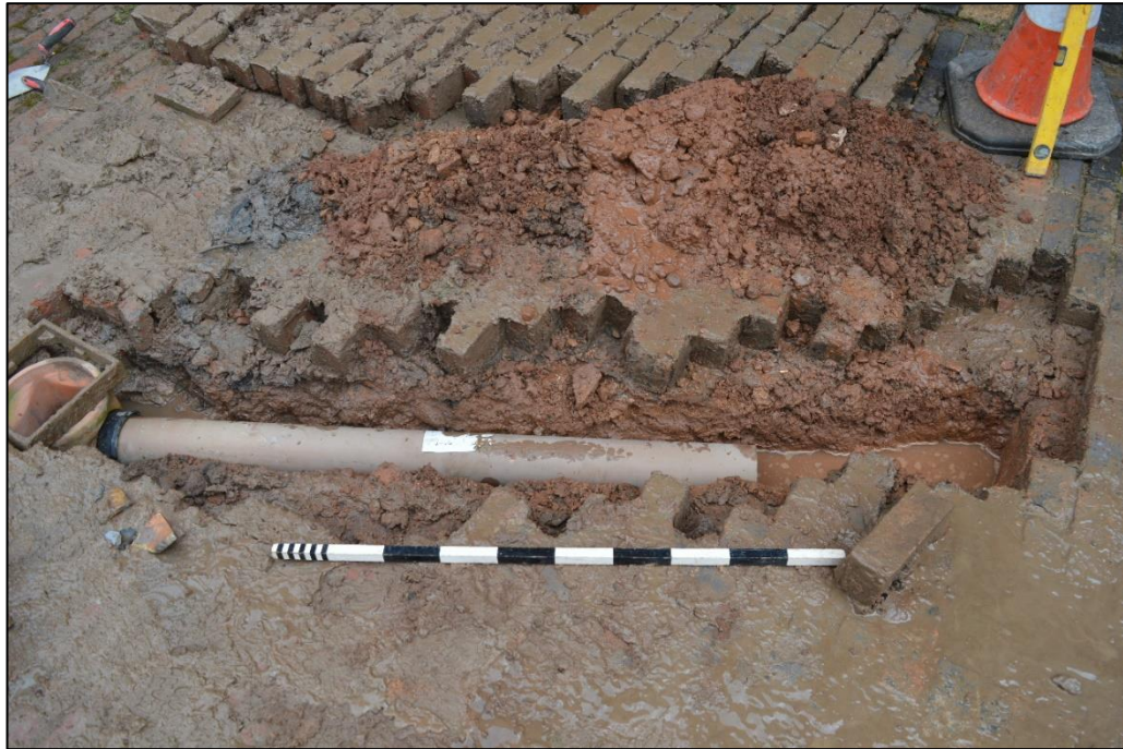
Fig. 3 View of the trenching from the south-west. Photo CPAT 4607-0001
