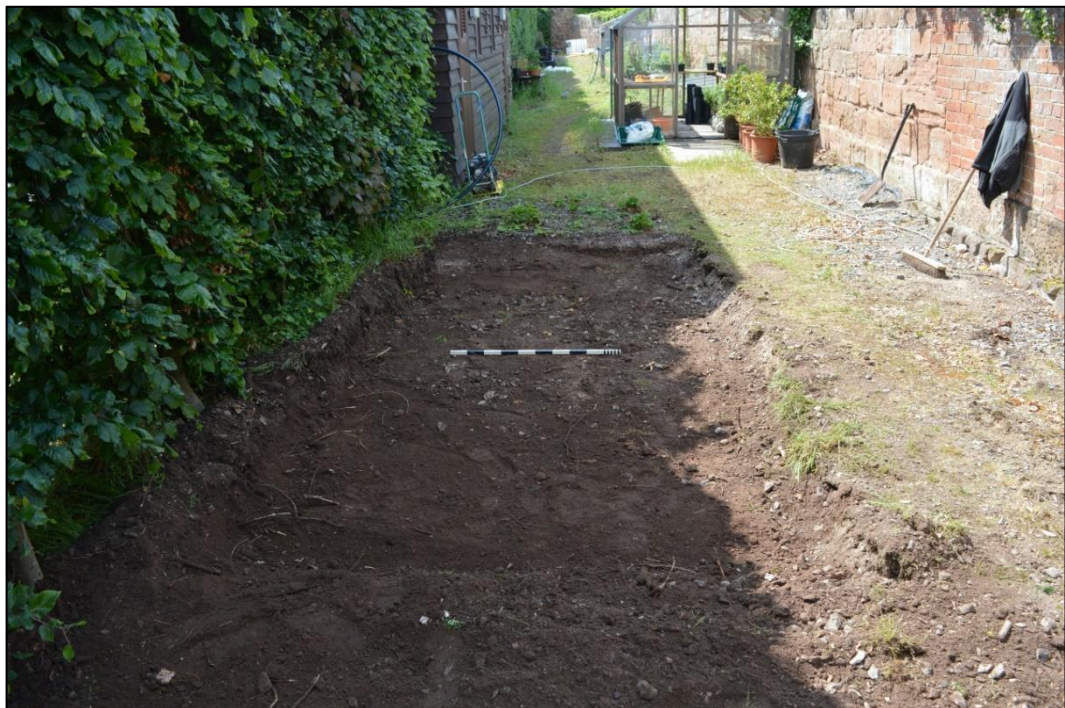
Fig. 3 Water tank trench viewed from the east. Photo CPAT 4649-009
