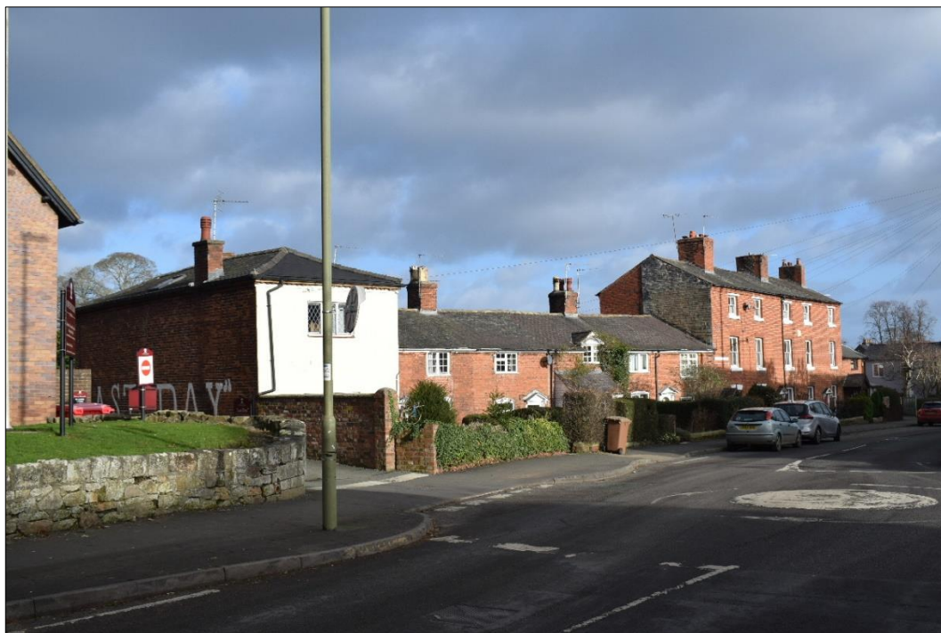
Fig. 16. View towards Oswestry Conservation Area with the 'Last Day Entrance' on the left. Photo CPAT 4582-0010
