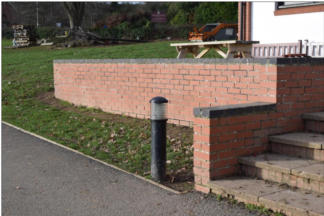
Fig. 11 The proposed lighting for the additional parking will be the same as that currently outside the cricket pavilion. Photo CPAT 4582-0014
