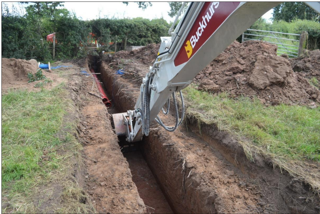
Fig. 5 Excavation of the cable trench. Photo CPAT 4700-0005
