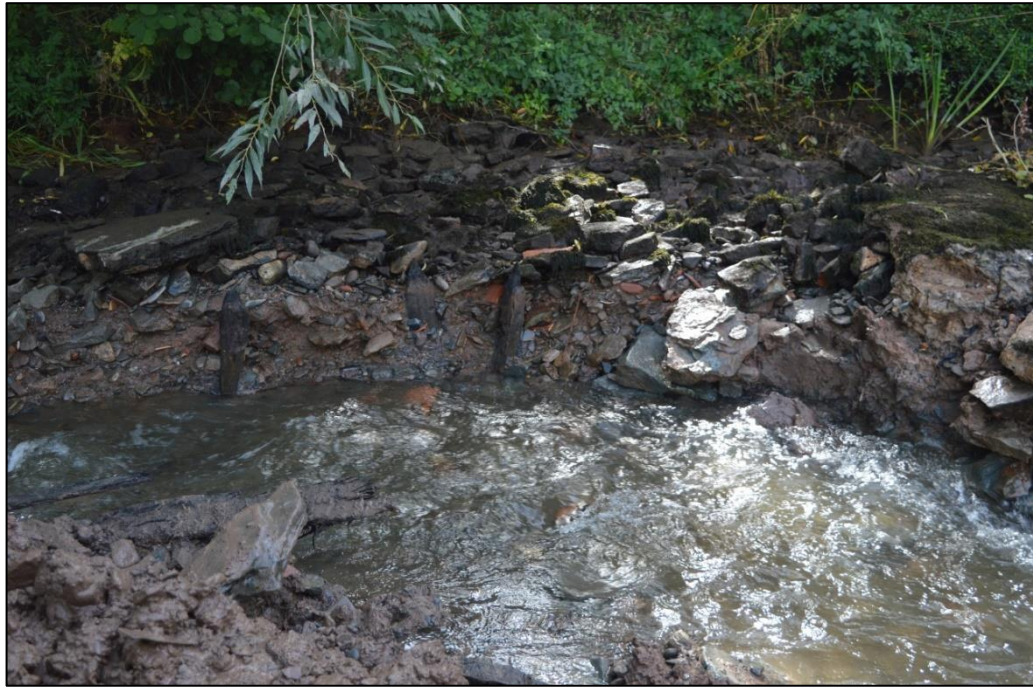
Fig. 12 View from the north-east showing the stakes used to retain the timber bracing Photo CPAT 4684-083
