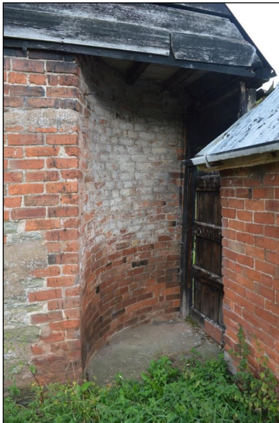
Fig. 8 Curved passageway on south-east corner of building Photo CPAT 4684-063
