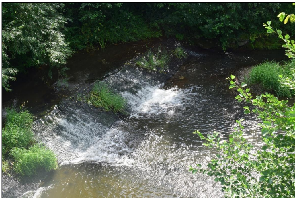
Fig. 2 The weir viewed from the north Photo CPAT 4684-030
