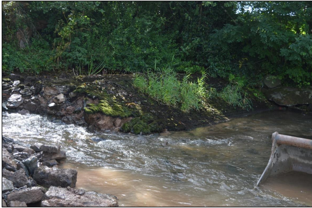
Fig. 10 The south-west end of the weir showing the smaller size of the setts used to construct this end of the structure Photo CPAT 4684-081
