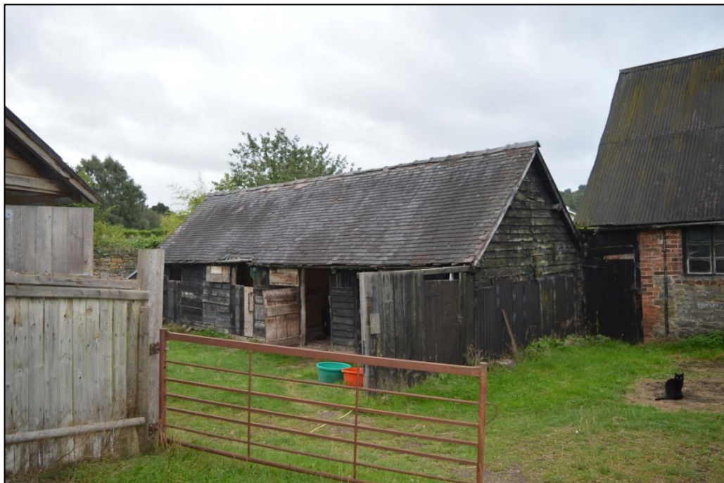
Fig. 6 South-eastern most building recorded on 1820 map, viewed from the north-east Photo CPAT 4684-072
