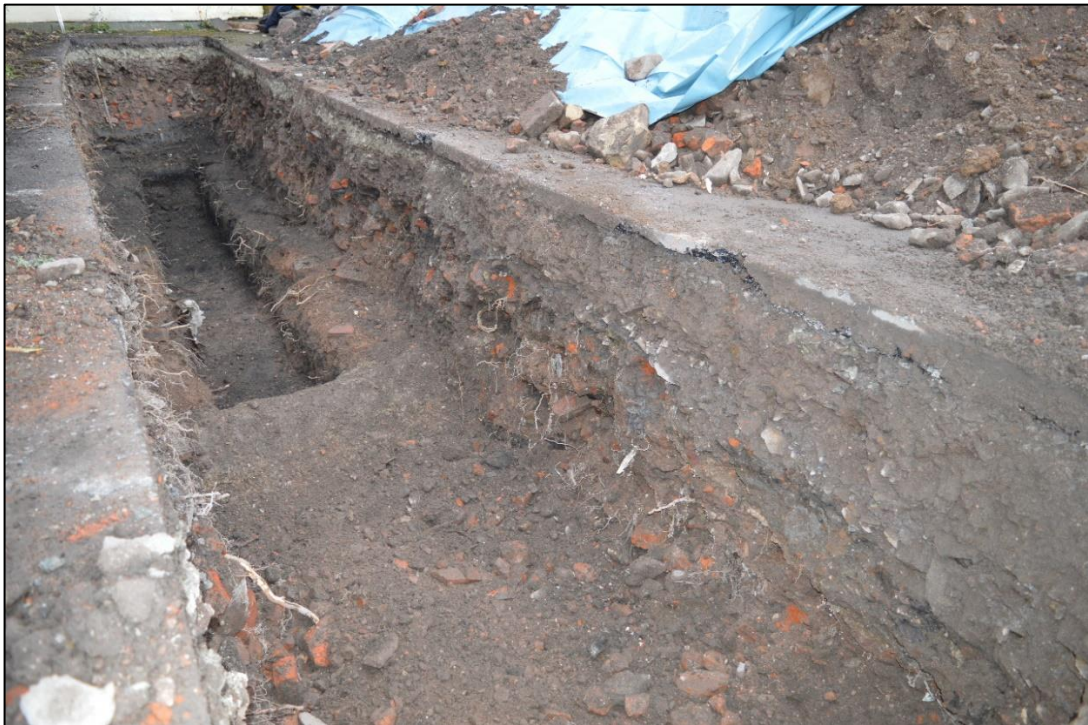
Fig. 14 Trench 2, viewed from the north-west. Photo CPAT 4470-0026
