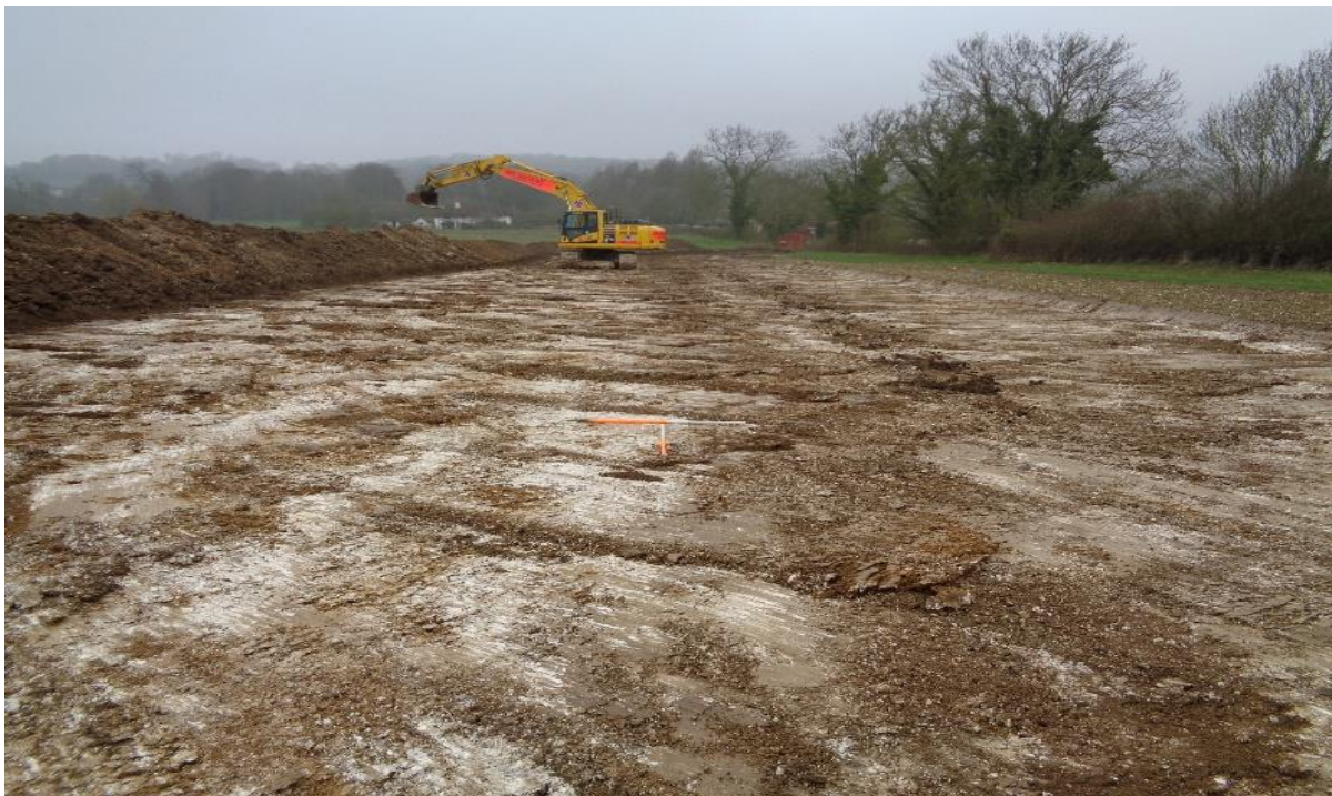
Plate 4: Trench 3 easement strip showing (003003) looking north-west (T-scale 1m x1m)
