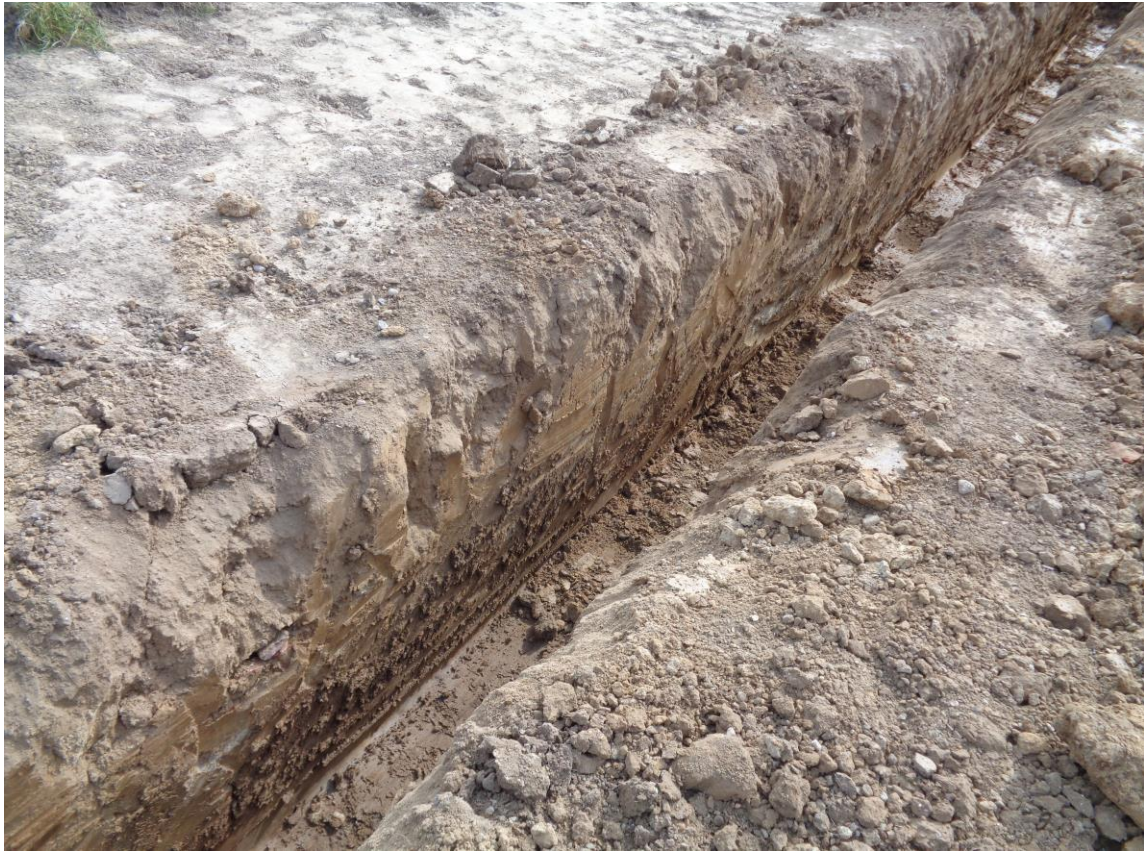
Plate 9: Trench 005 showing natural substrate (005003) in E-facing section of pipe-trench
