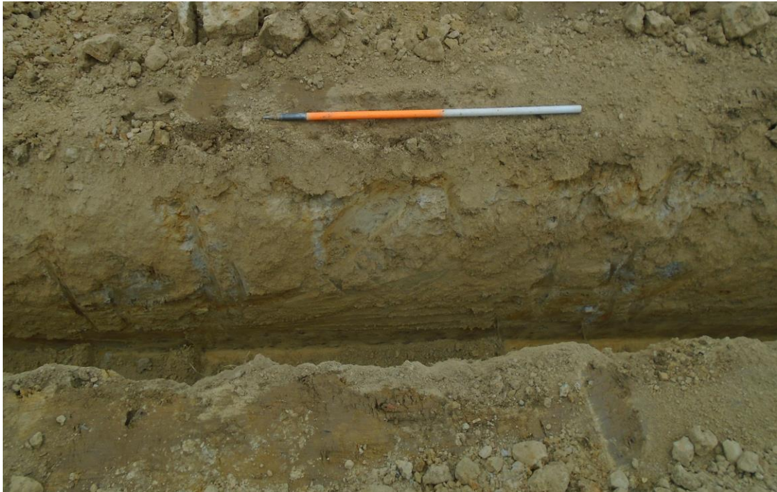
Plate 7: Trench 003, pipe-trench showing south-facing section, looking N (1m scale)
