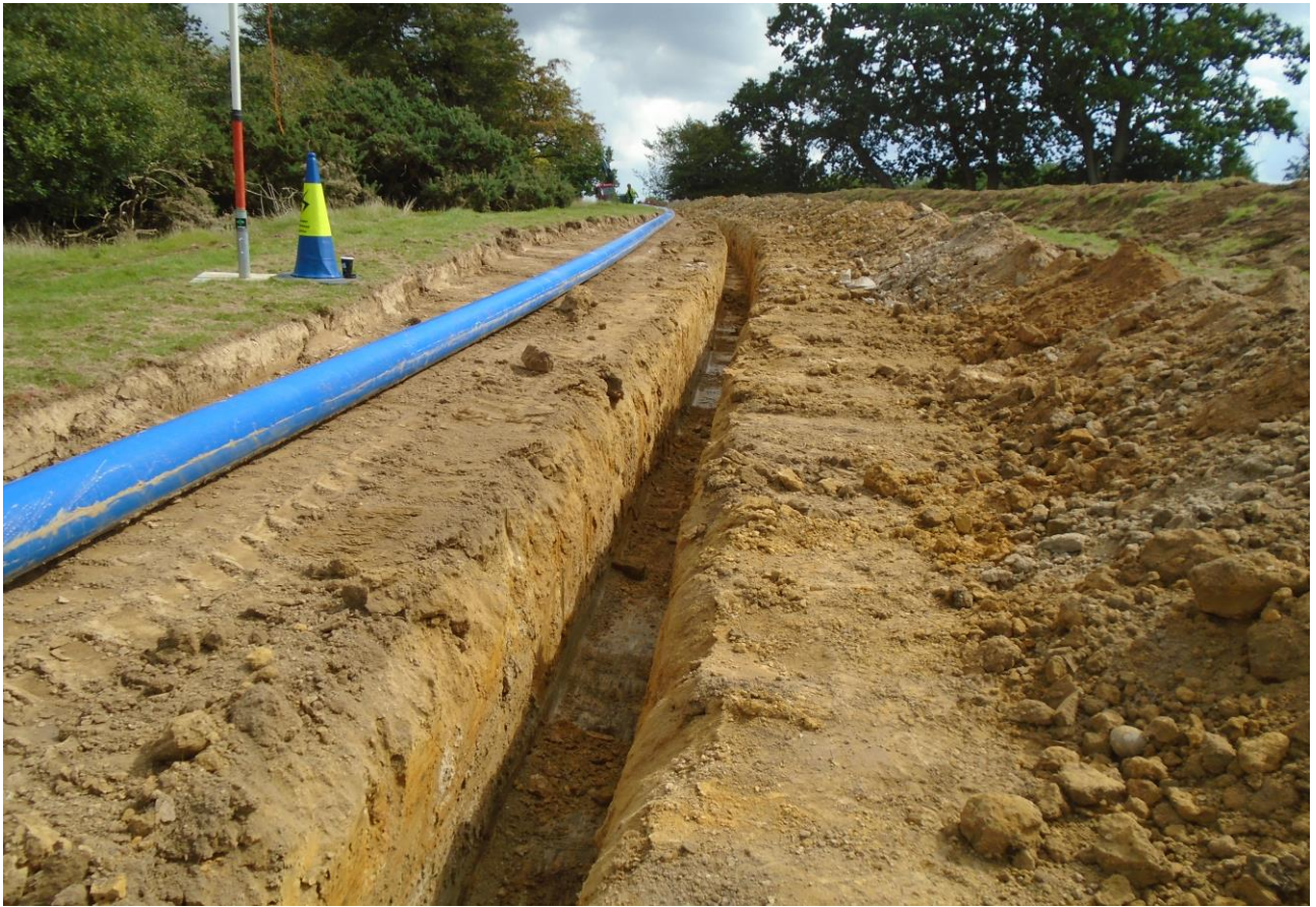
Plate 3: Pipe-trenching in Trench 001, looking ESE
