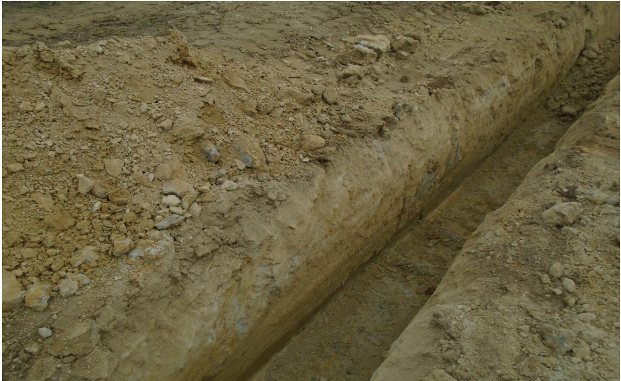
Plate 5: S-facing section showing natural substrate (002003) within the pipe-trench in Trench 002, looking ENE
