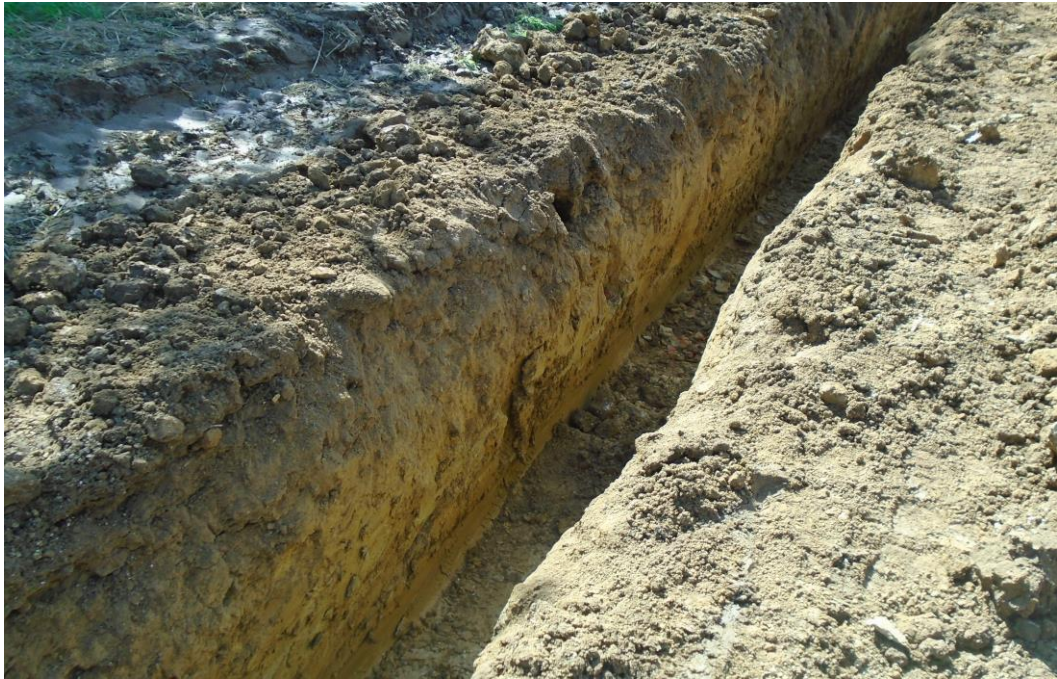
Plate 8: Trench 004 pipe-trench showing subsoil (004002) and natural substrate (004003), looking SSE
