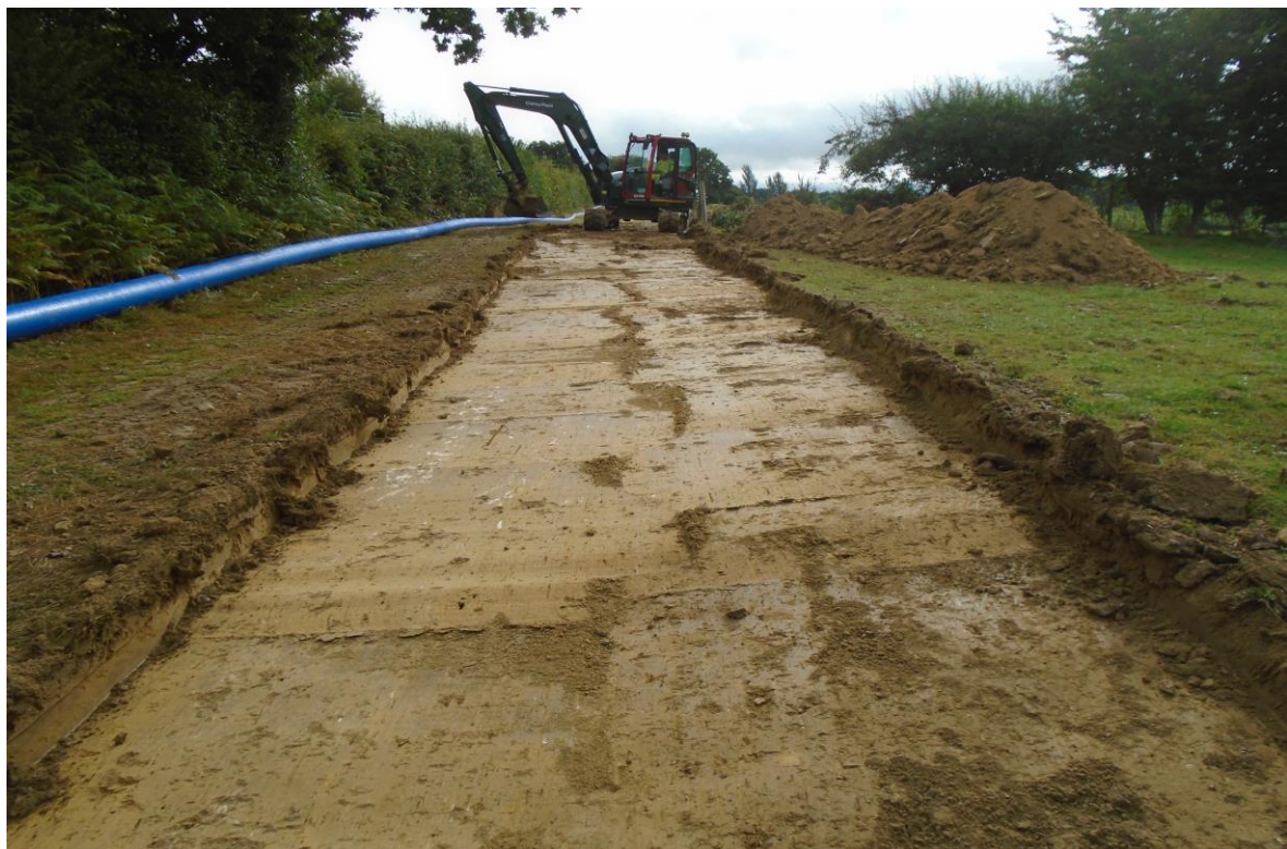
Plate 4: General view of topsoil strip in Trench 002 showing subsoil (002002), looking ESE
