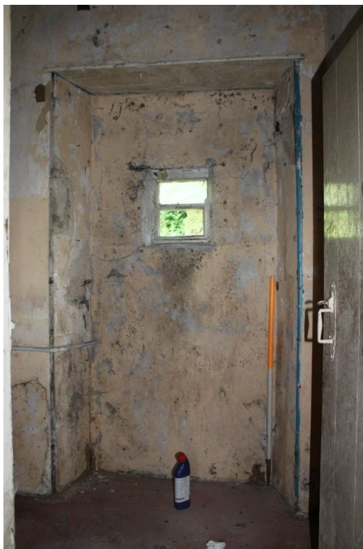
Plate 32: internal view NNW within ground toilet room, showing sash window within blocked up doorway – Building No. 1
