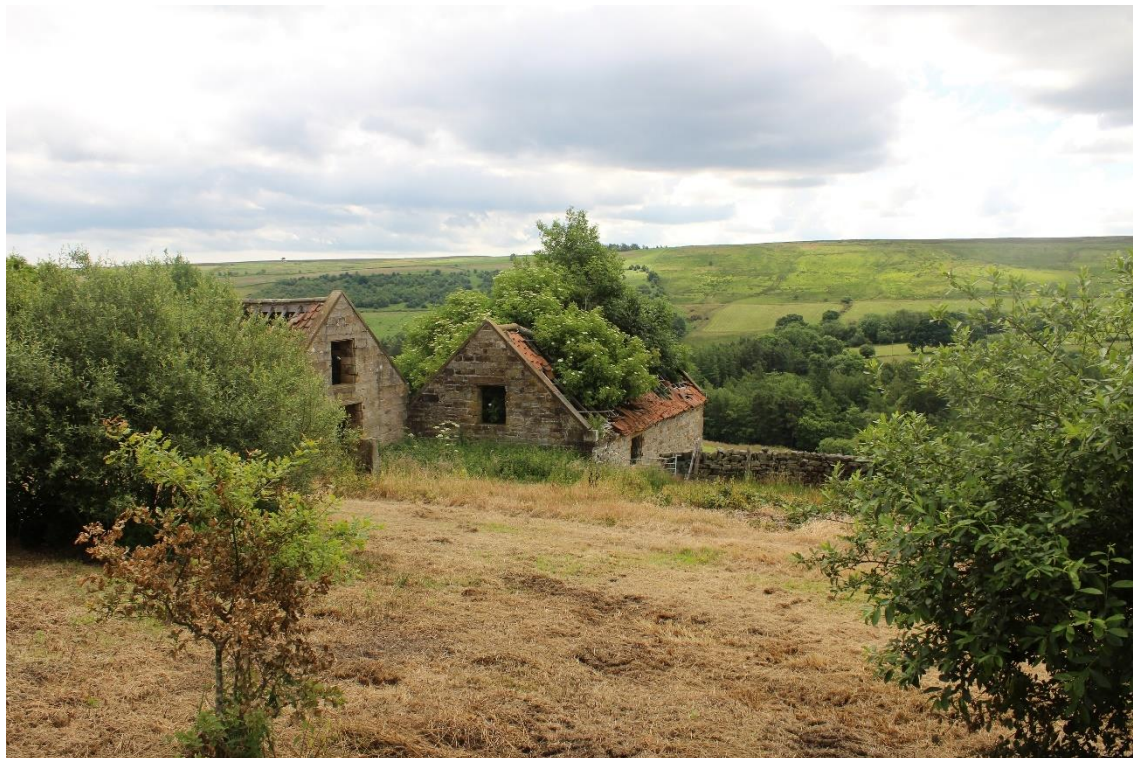
Plate 109: Oblique view ESE of Buildings No. 2 & 3
