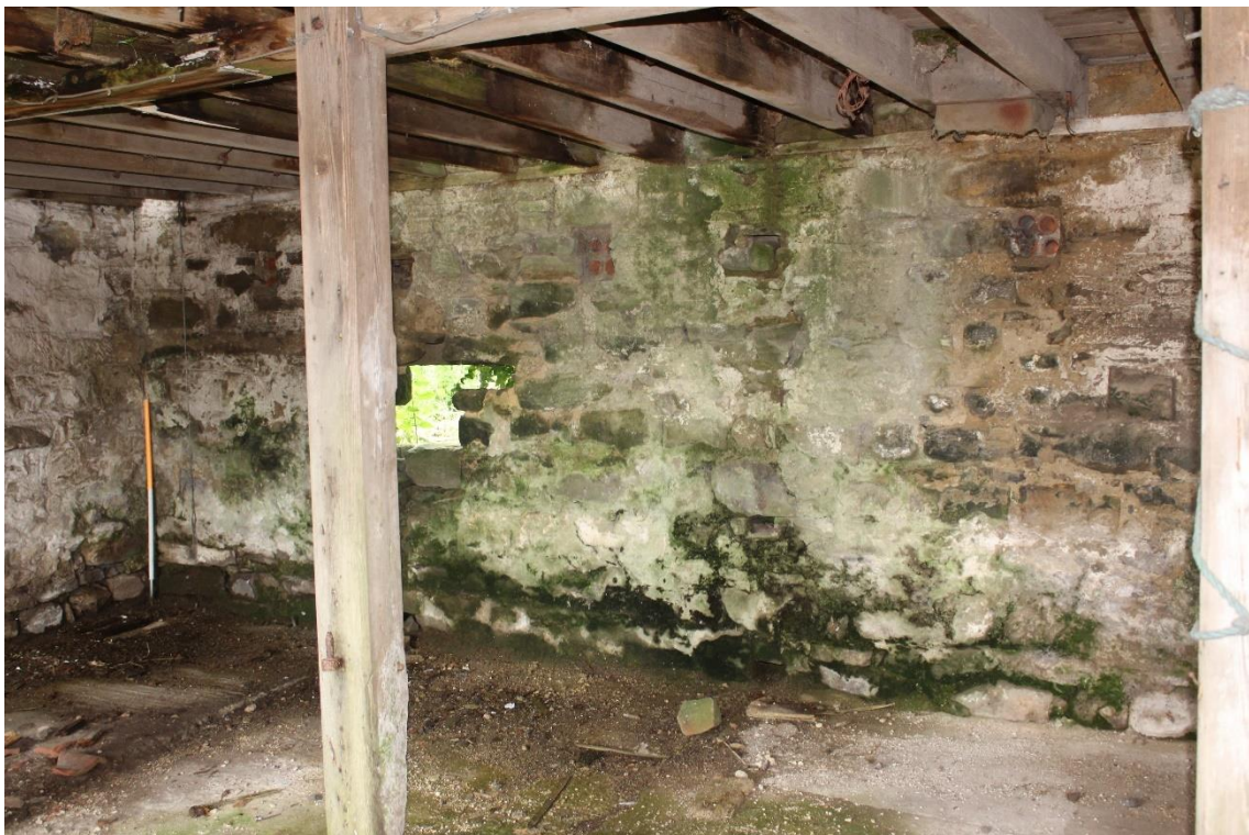
Plate 128: Internal view NW of the first compartment of Building No.4
