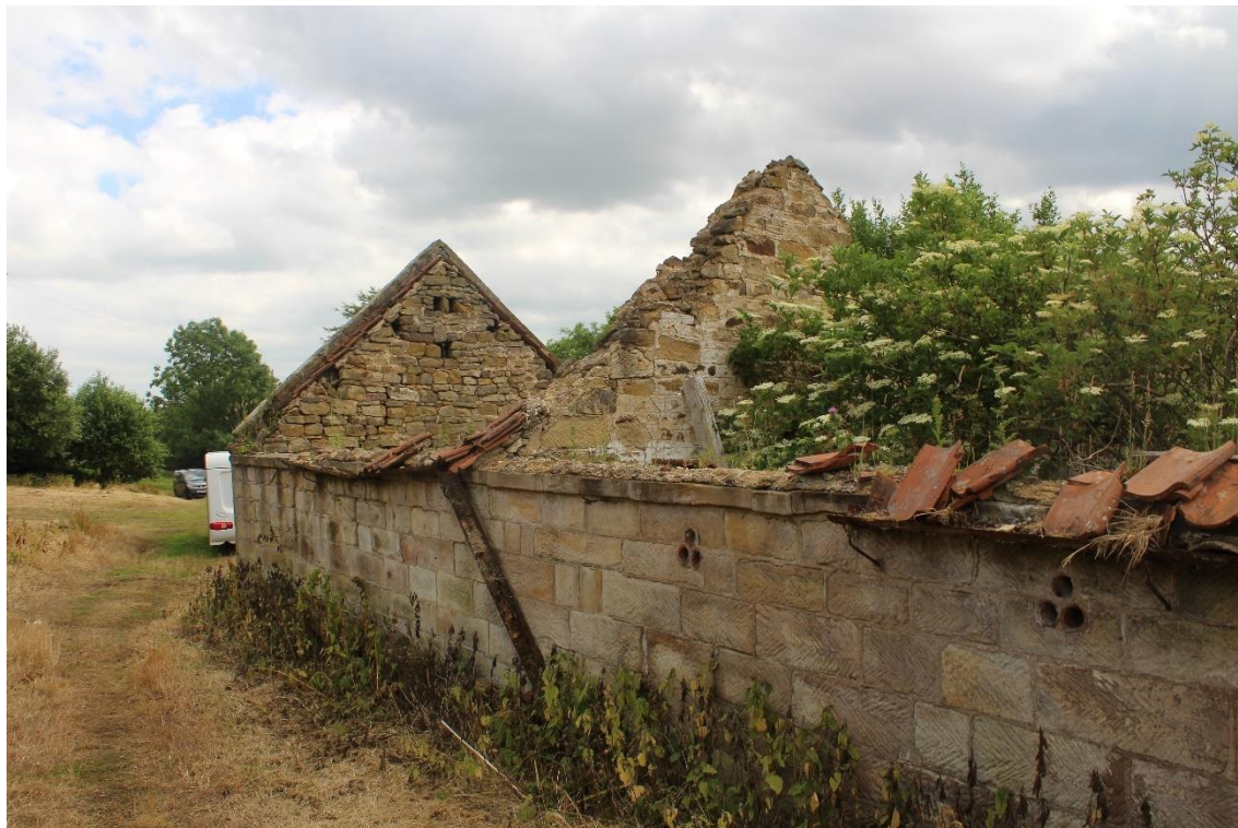
Plate 103: External oblique view of N-facing elevation of Building No. 2
