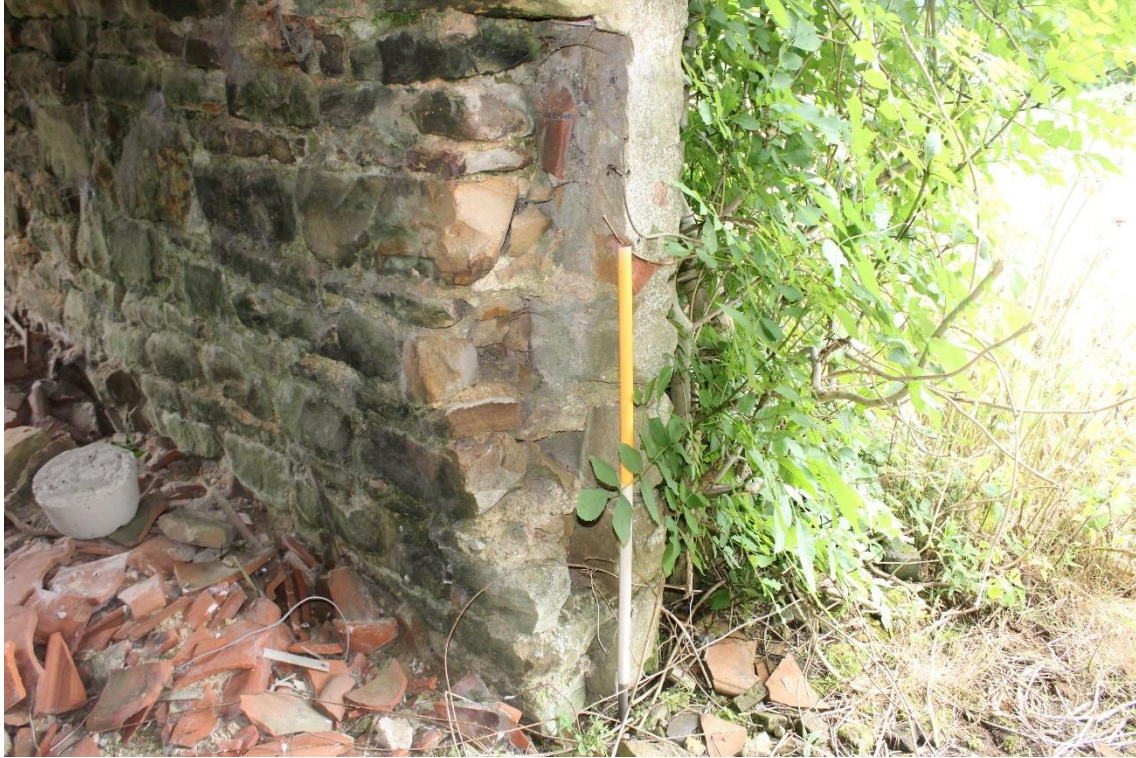
Plate 151: Internal view SE showing wall construction within the third compartment of Building No.4
