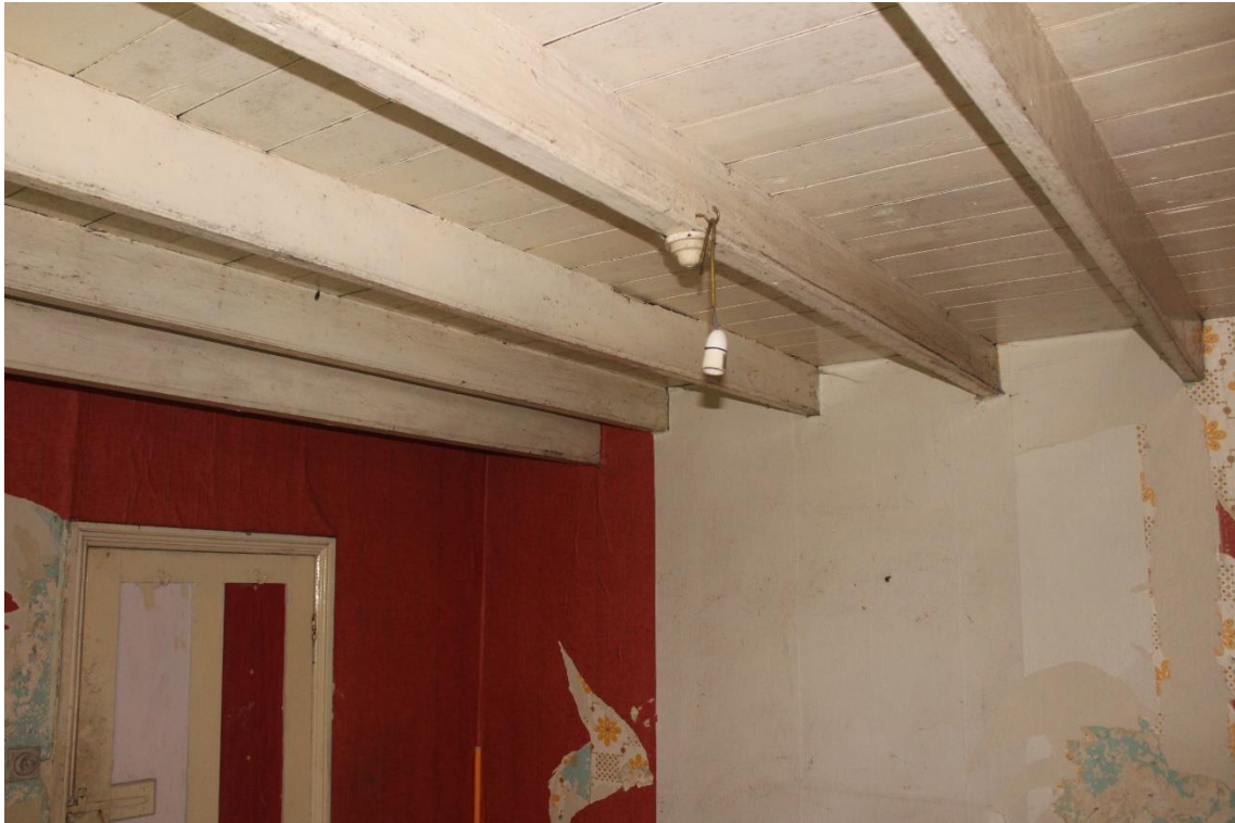
Plate 73: Internal view SE of 1 st floor second bedroom showing ceiling – Building No.1
