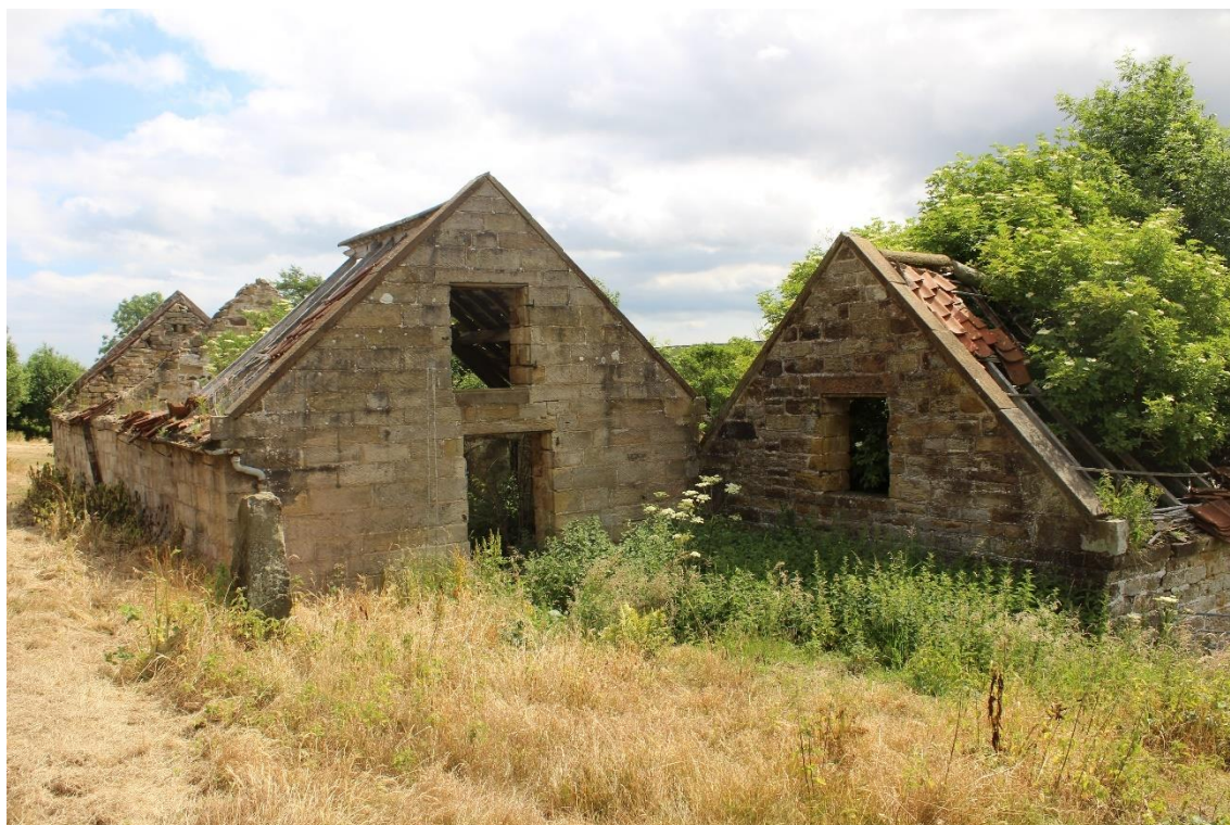
Plate 106: Oblique view ESE of Buildings No. 2 & 3
