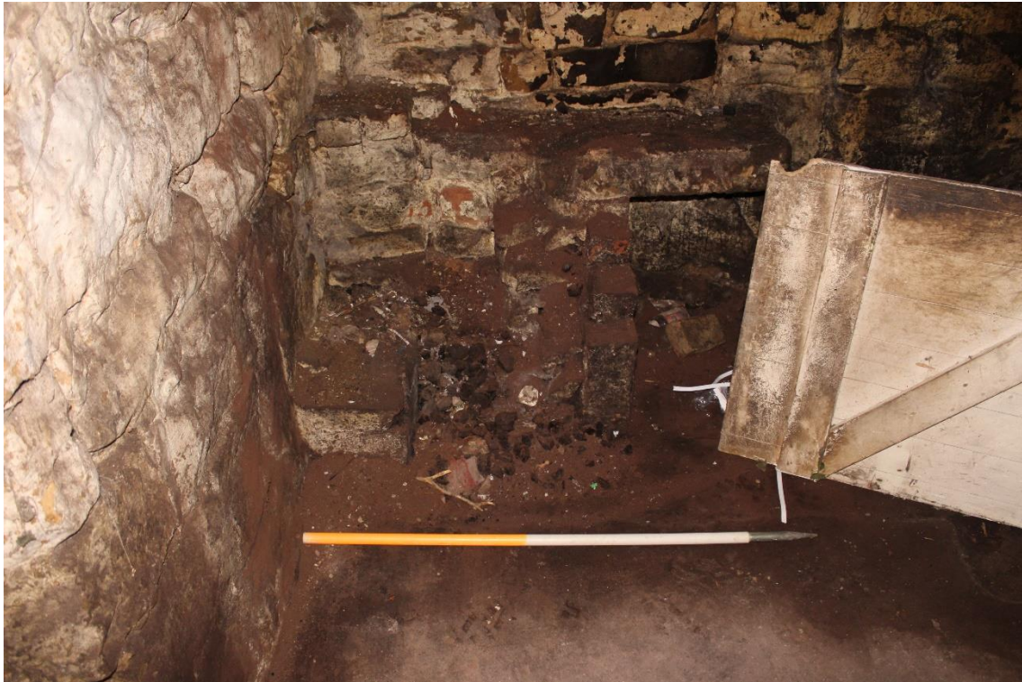
Plate 49: internal view WSW within ground floor outhouse showing stove – Building No. 1
