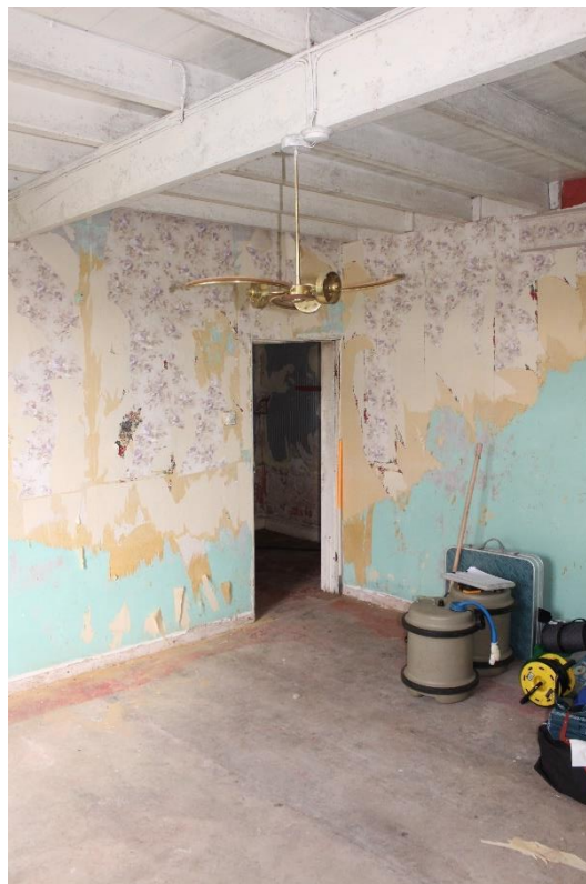
Plate 40: internal view SE within ground sitting room – Building No. 1
