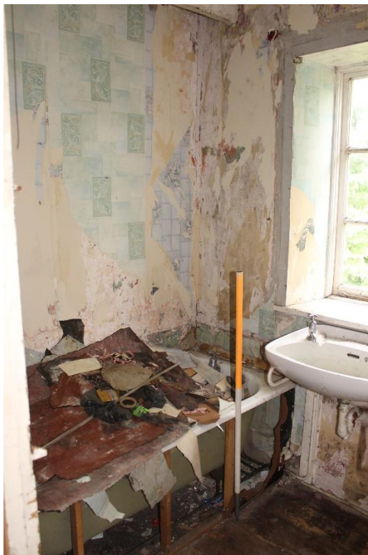
Plate 74: Internal view NW of 1 st floor bathroom – Building No.1
