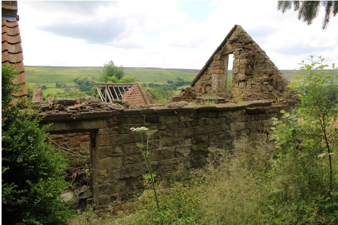
Plate 11: View SSW showing N facing elevation of pigsty (Building No. 1)
