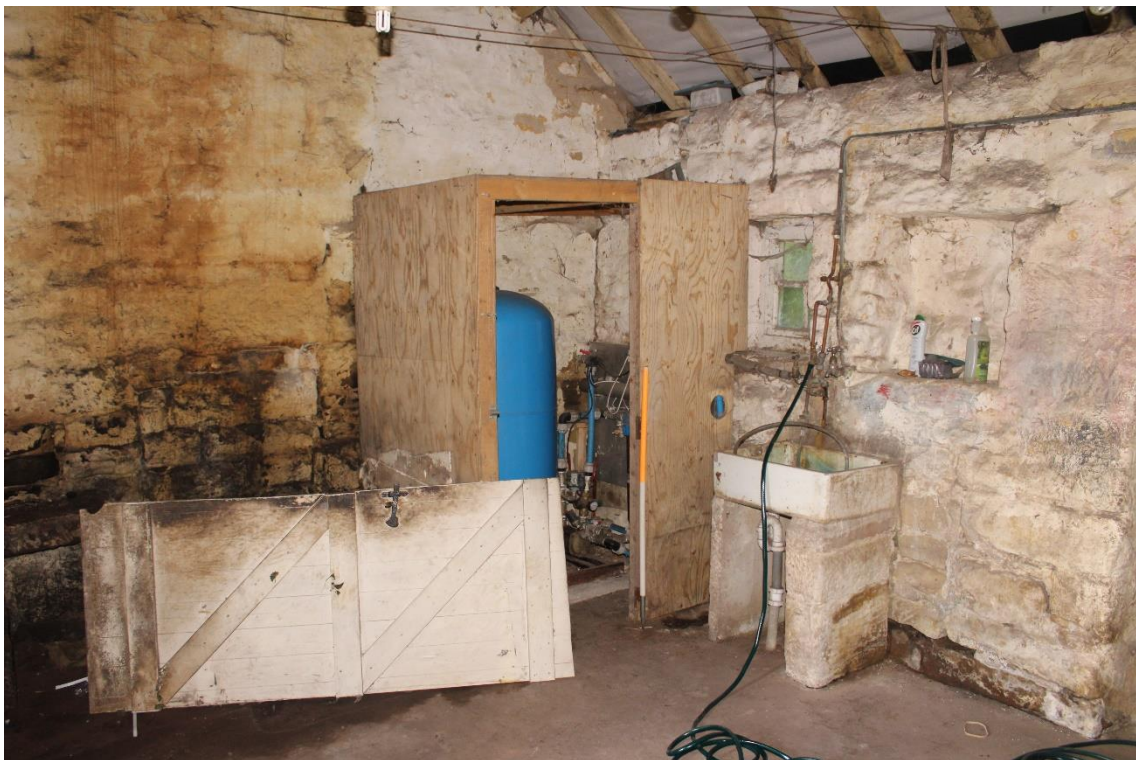
Plate 44: internal view NW within ground floor outhouse – Building No. 1
