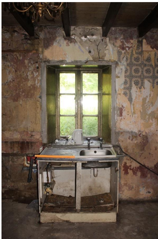
Plate 29: internal view NNW within ground floor kitchen showing casement window – Building No. 1
