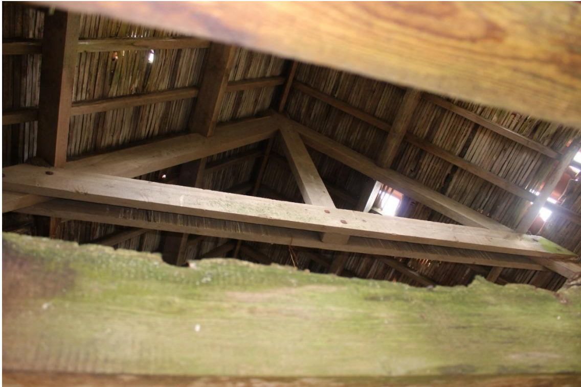
Plate 133: Internal view ESE of king post roof truss within the first compartment of Building No.4
