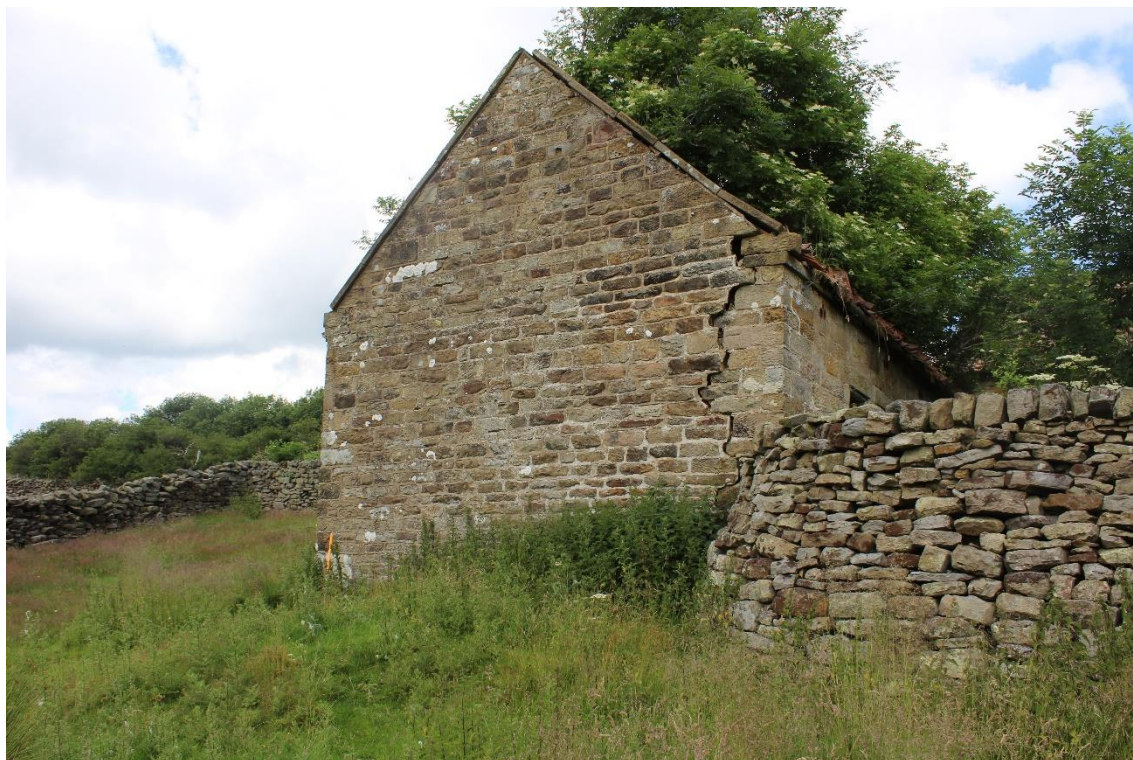
Plate 115: External view NW of S and E-facing elevations of building No.3
