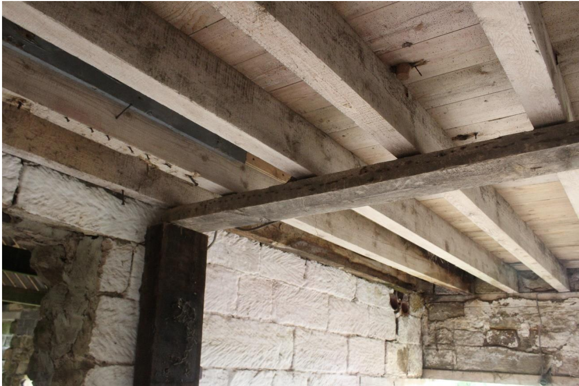
Plate 141: Internal view SSE of the roof timbers within the second compartment of Building No.4
