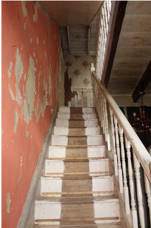
Plate 15: Internal view NNW showing ground floor staircase within the farmhouse – Building No. 1
