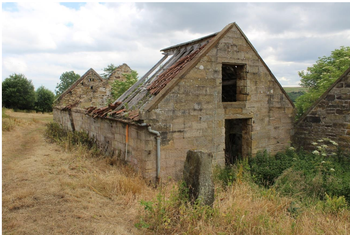
Plate 105: Oblique view ESE of N and W-facing elevation of Building No. 2
