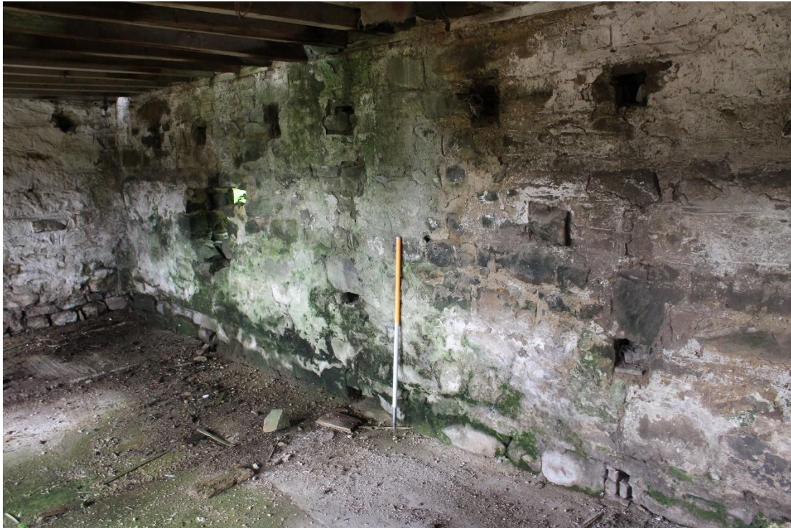
Plate 135: Internal view NW showing fixtures on the N wall aligned with the struts within the first compartment of Building No.4
