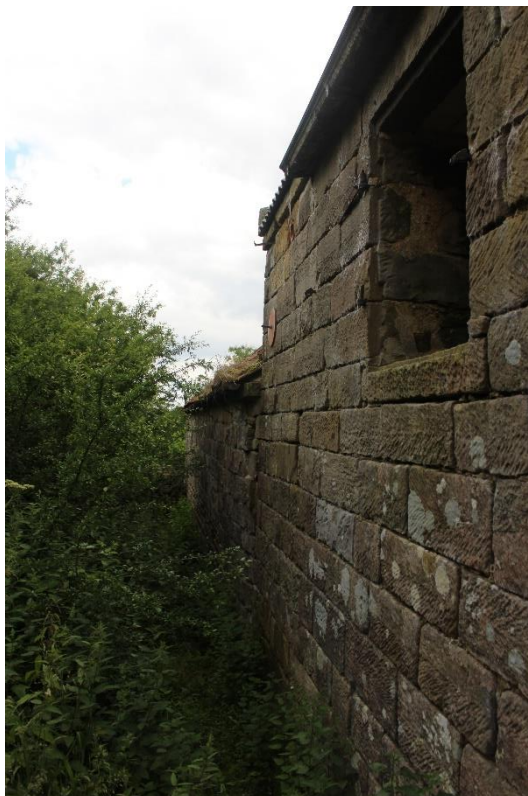
Plate 126: Oblique external view ESE of N-facing elevation of Building No.4
