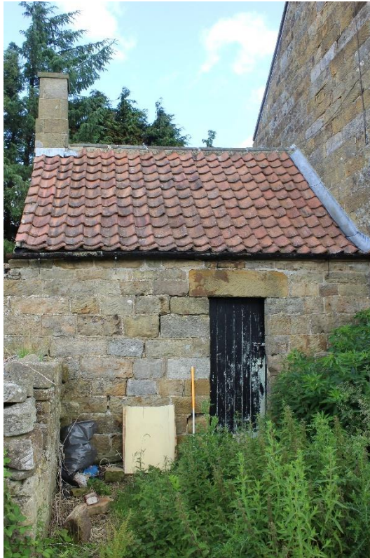
Plate 95: External view NNW of outhouse of Building No. 1
