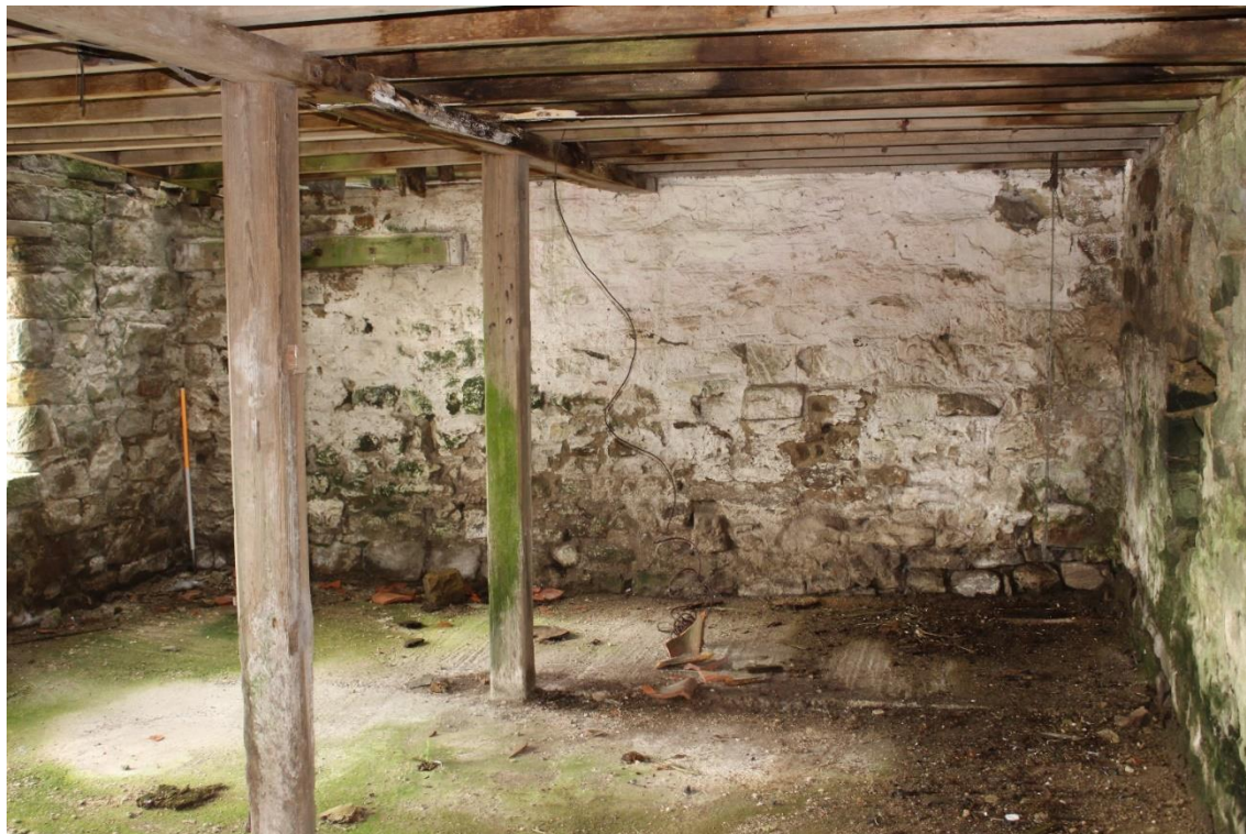
Plate 129: Internal view WSW of the first compartment of Building No.4
