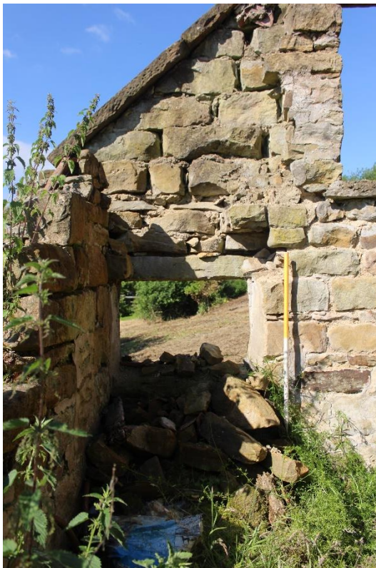
Plate 53: internal view WSW of pigsties W partition showing blocked doorway— Building No. 1
