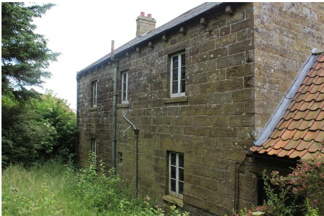
Plate 8: View ESE showing N facing elevation of the farmhouse Building No. 1
