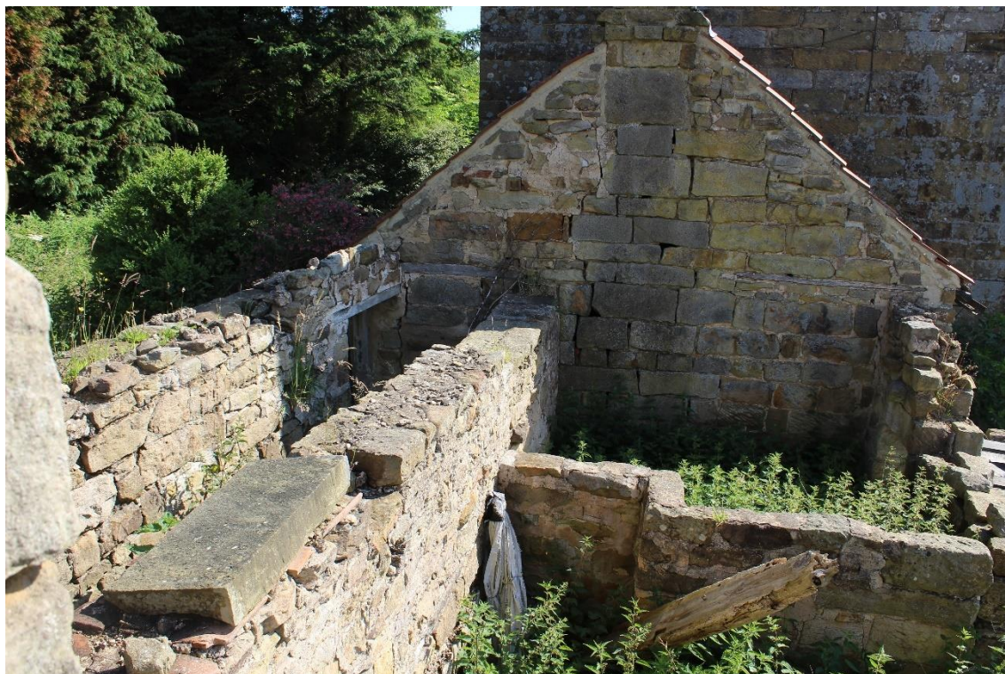
Plate 56 internal view W of pigsties W – Building No. 1
