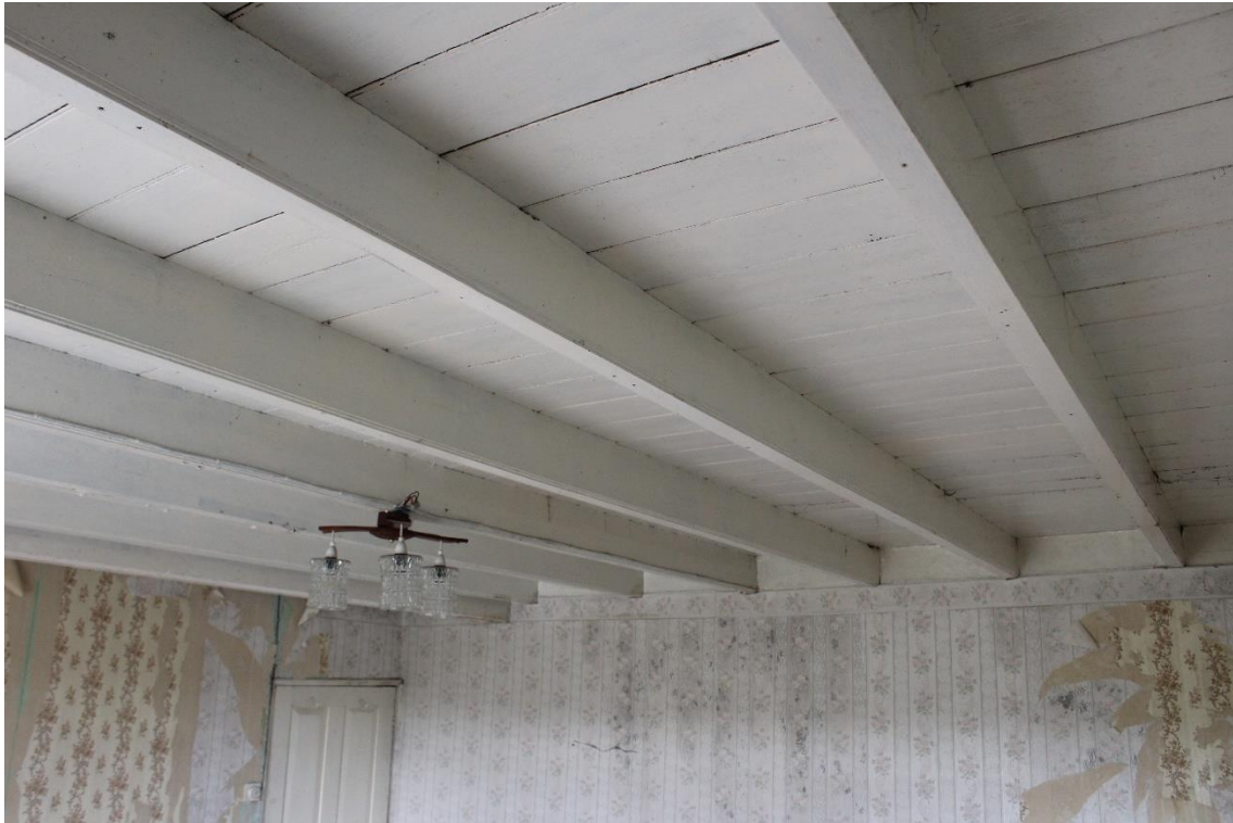
Plate 85: Internal view WSW of 1 st floor fourth bedroom showing ceiling – Building No.1
