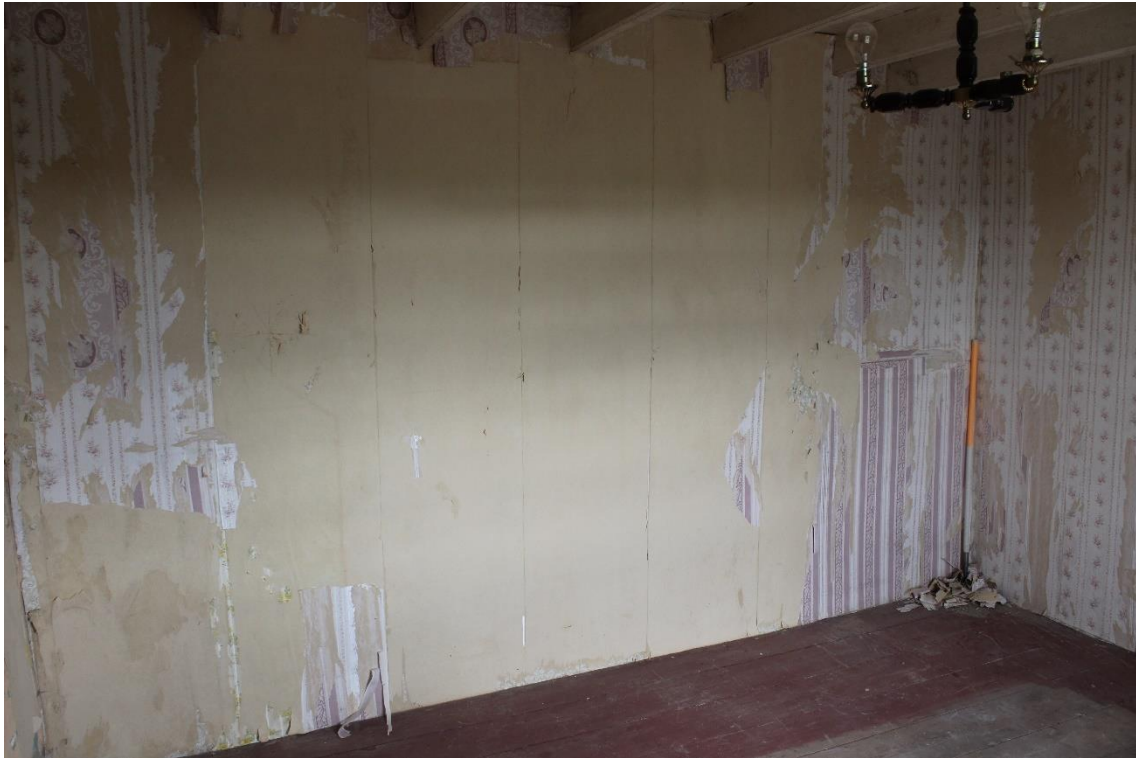
Plate 67: Internal view NE of 1 st floor bedroom – Building No.1
