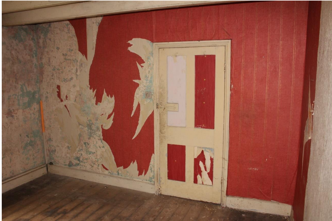
Plate 71: Internal view NE of 1 st floor second bedroom – Building No.1
