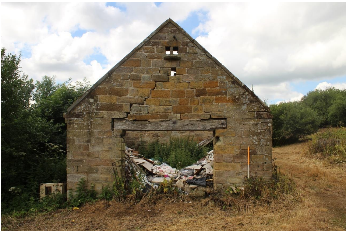
Plate 98: Exterior view WSW of the E elevation of Building No. 2
