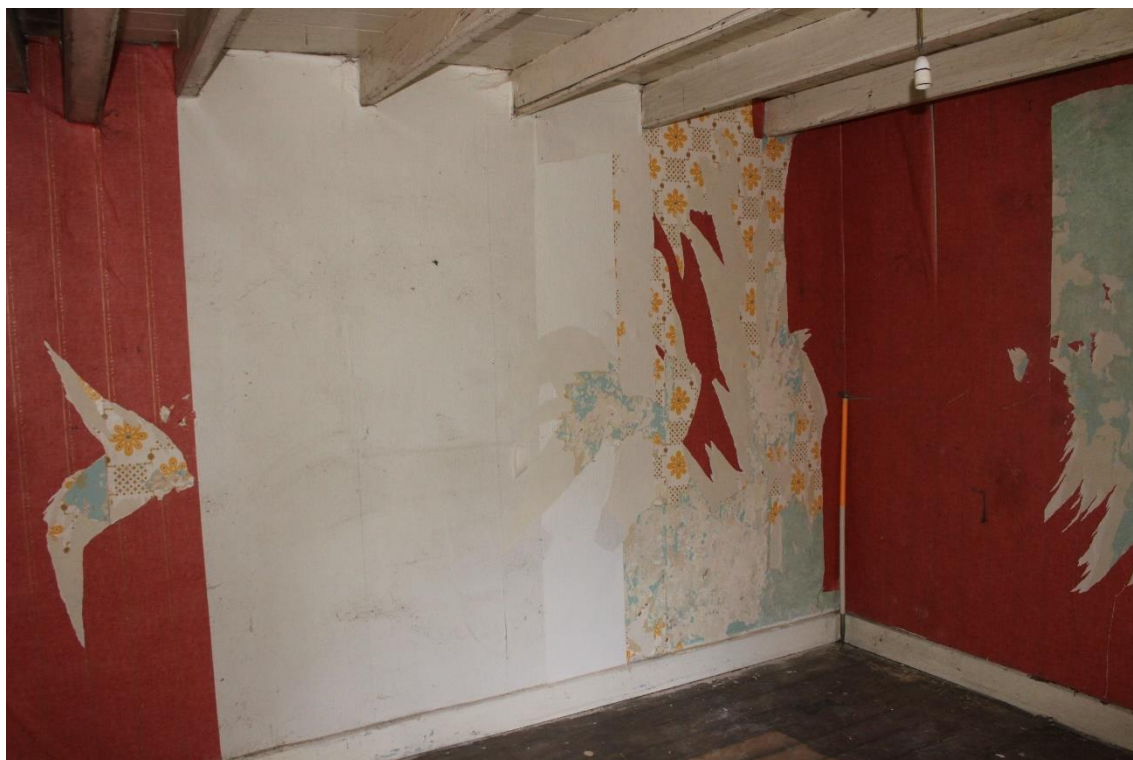
Plate 70: Internal view SW of 1 st floor second bedroom – Building No.1
