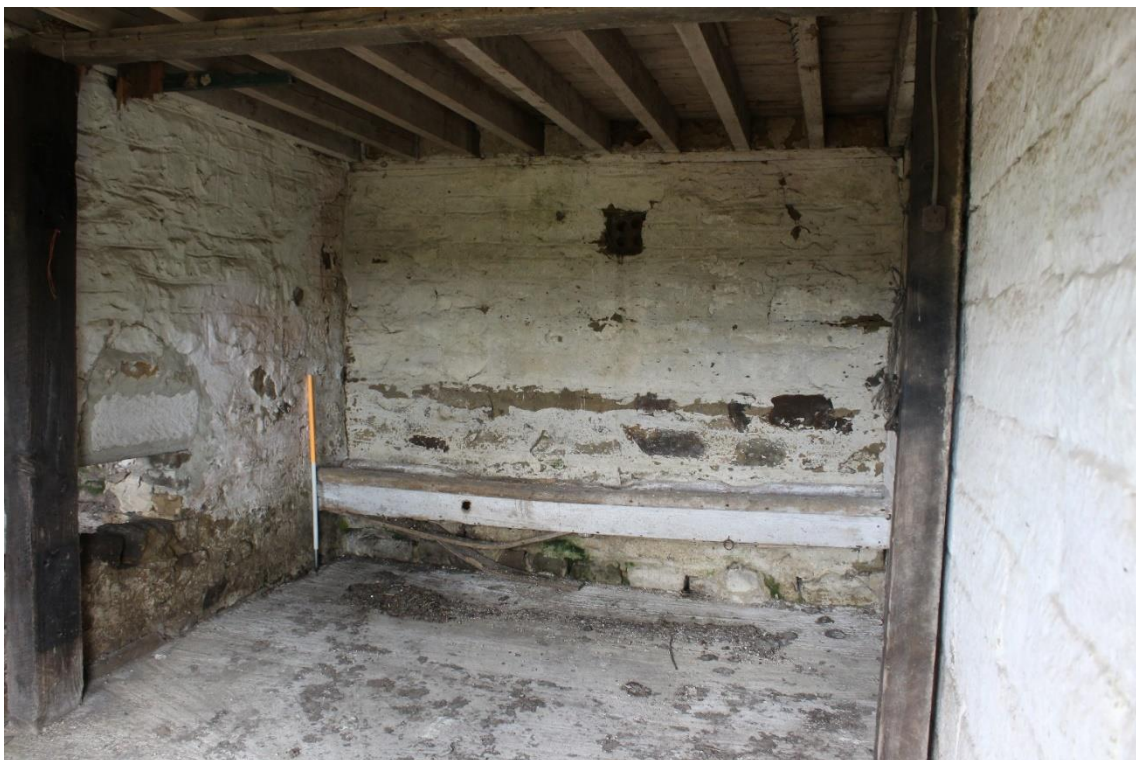
Plate 136: Internal view NNW of the second compartment of Building No.4
