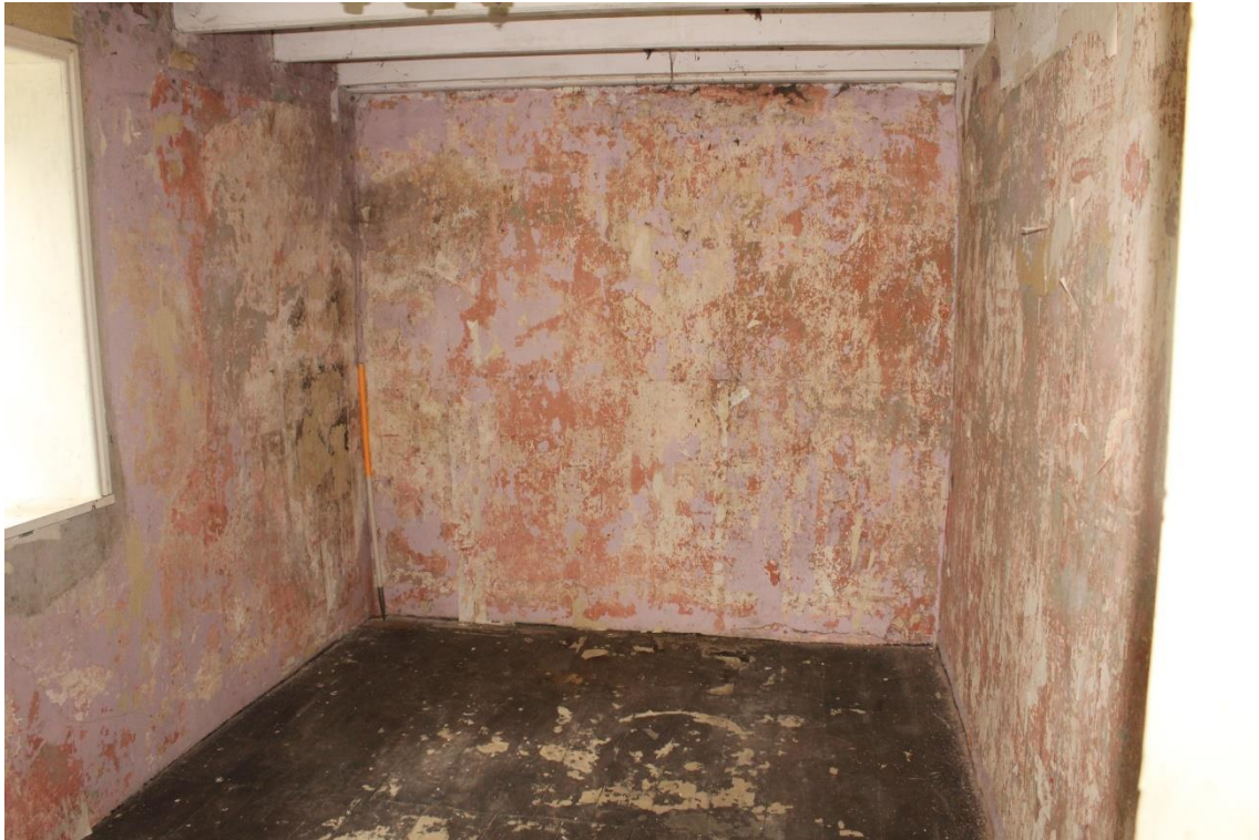
Plate 77: Internal view ENE of 1st floor third bedroom – Building No.1
