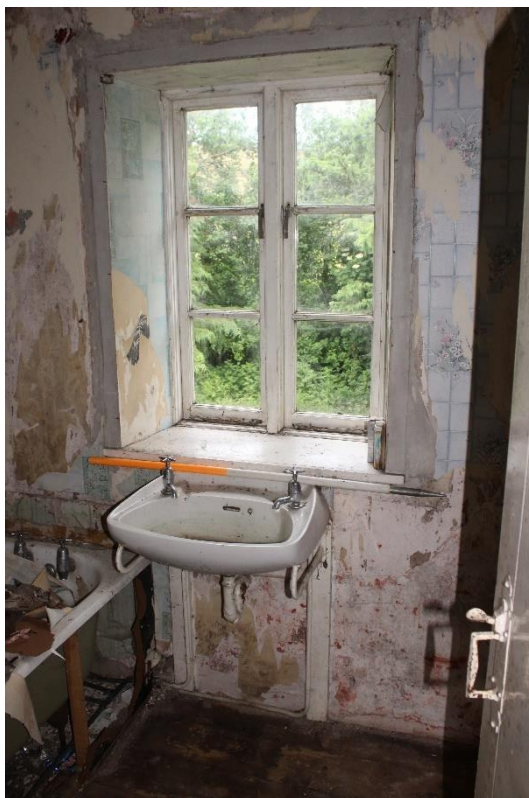
Plate 75: Internal view NNW of 1 st floor bathroom showing two light casement window within N wall – Building No.1
