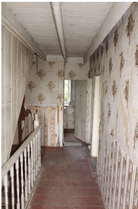
Plate 62 Internal view NNW of 1 st floor central hall way – Building No.1
