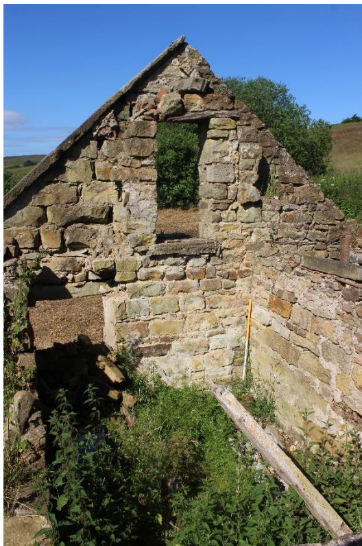
Plate 52: internal view W of pigsties W partition – Building No. 1
