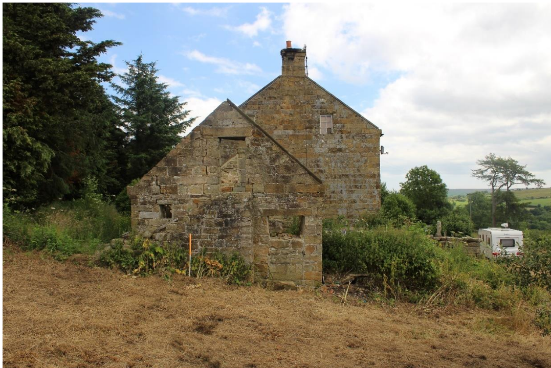
Plate 5: View ENE showing W facing elevation of Building No. 1, including the pigsty (foreground) and the farmhouse (background)
