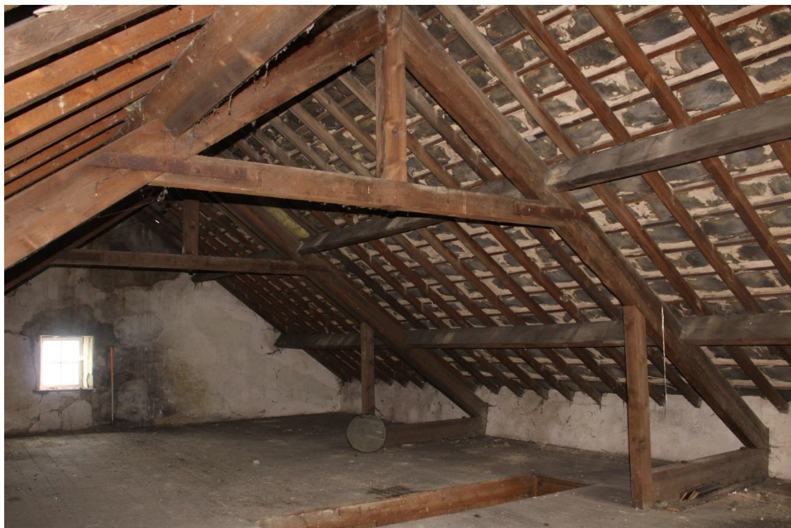
Plate 90: Internal view E of attic/roof space showing roof trusses – Building No.1
