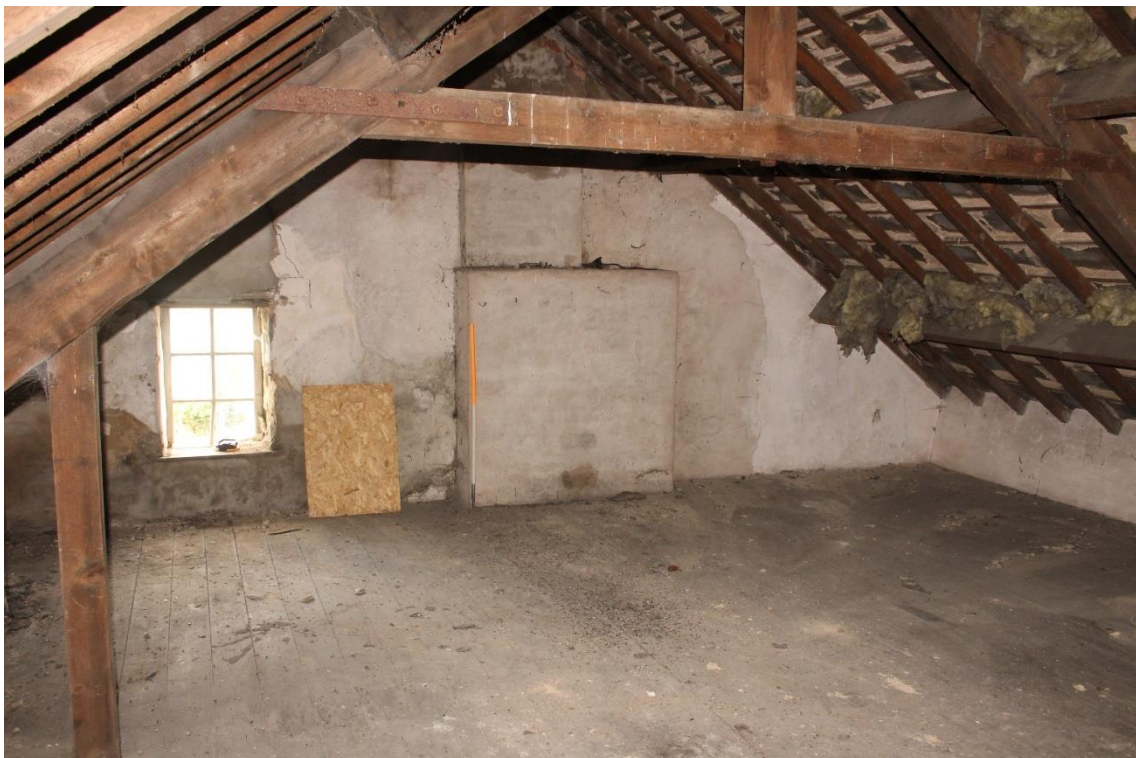
Plate 92: Internal view ENE of attic/roof space showing blocked fireplace and single light casement window – Building No.1
