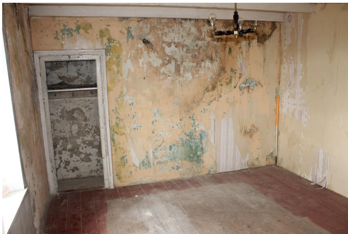
Plate 64: Internal view W of 1 st floor bedroom— Building No.1
