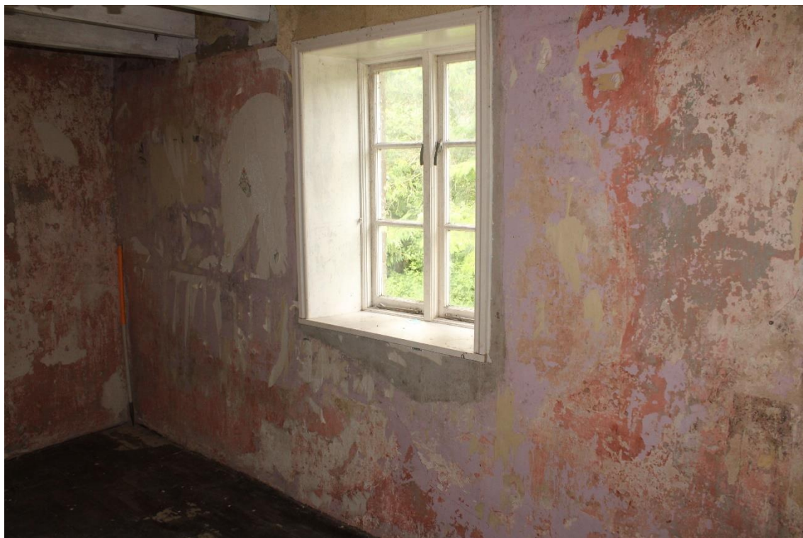
Plate 79: Internal view NW of 1 st floor third bedroom showing two light casement window with N wall – Building No.1
