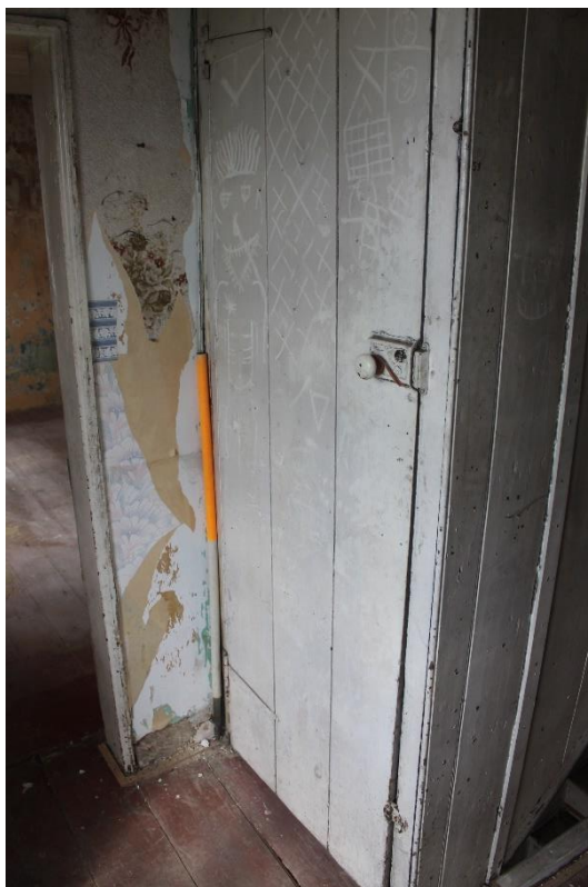
Plate 63: Internal view NW of 1 st floor central hall way showing attic stairs entrance— Building No.1
