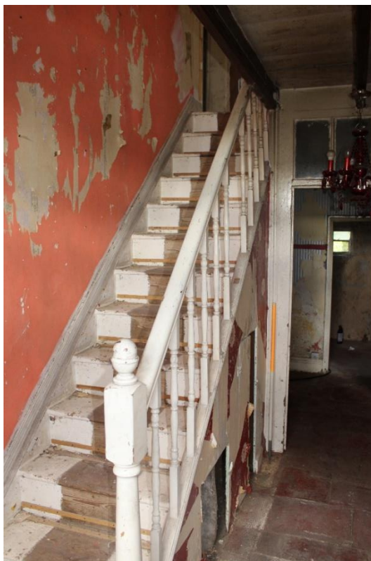
Plate 14: Internal view NW showing ground floor staircase within the farmhouse – Building No. 1
