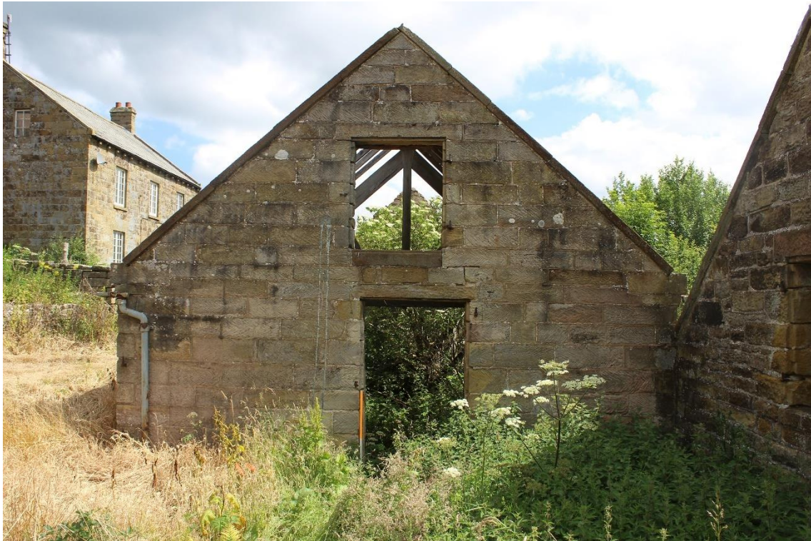
Plate 107: External view ENE of W-facing gable end of Building No.2
