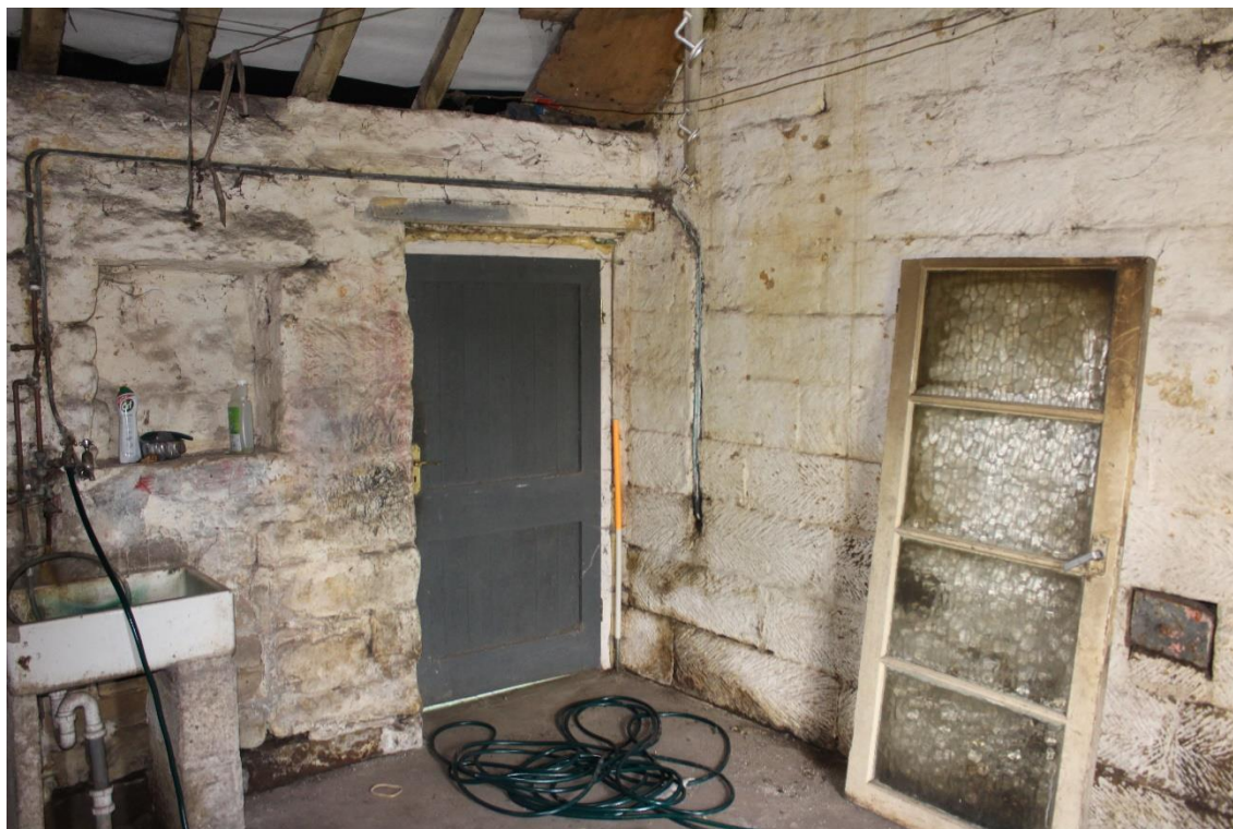
Plate 47: internal view NE within ground floor outhouse – Building No. 1
