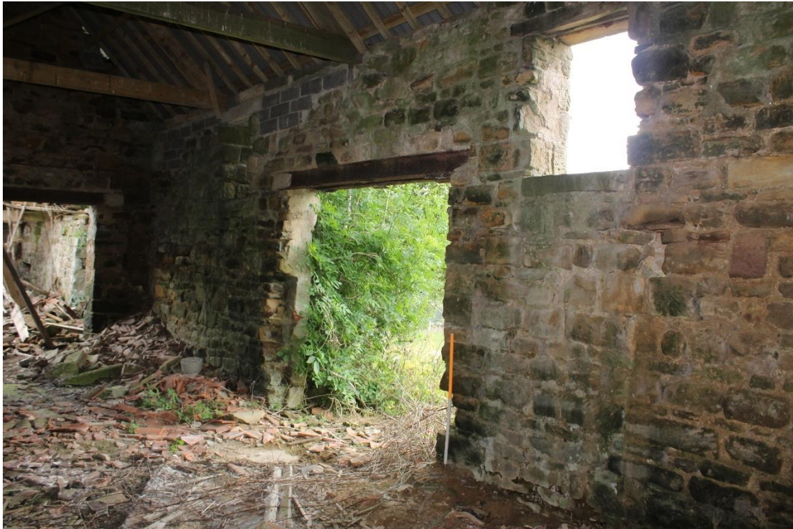
Plate 149: Internal view SE of the third compartment of Building No.4
