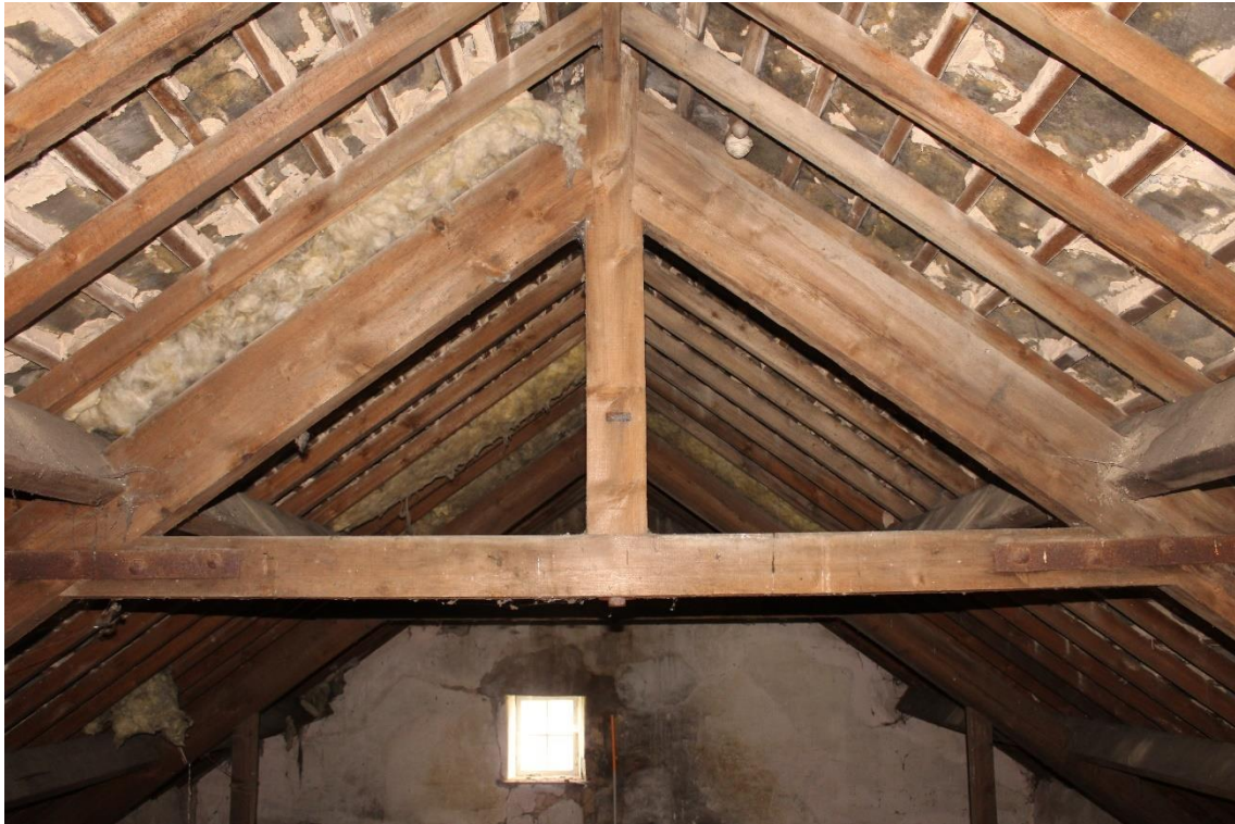
Plate 93: Internal view ENE of attic/roof space showing rood timbers – Building No.1
