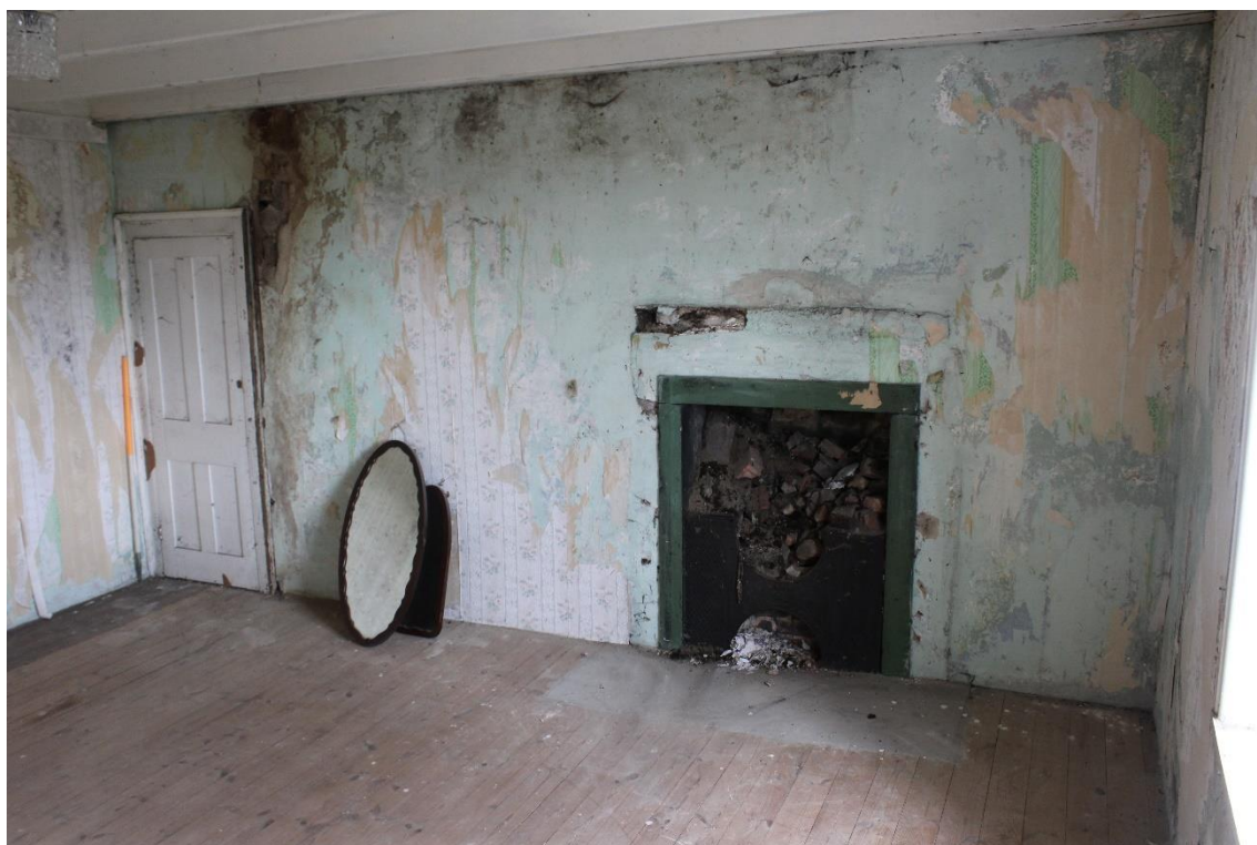
Plate 82: Internal view NE of 1 st floor fourth bedroom showing fireplace and locked storage alcove– Building No.1
