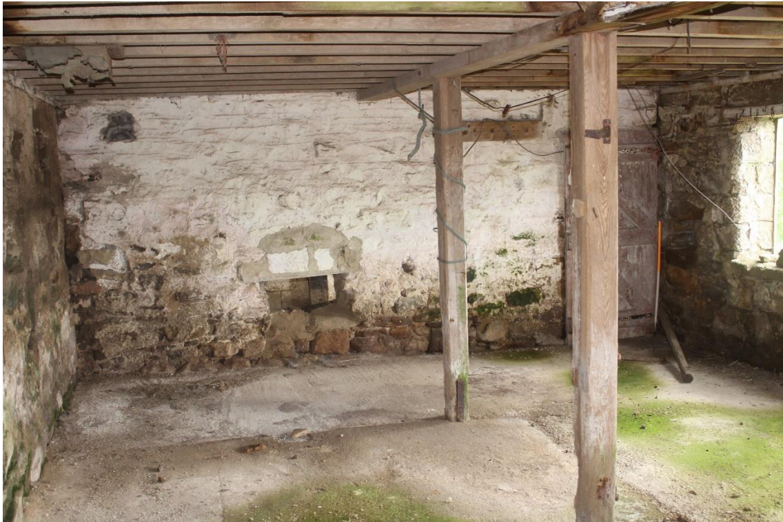
Plate 127: Internal view ESE of the first compartment of Building No.4
