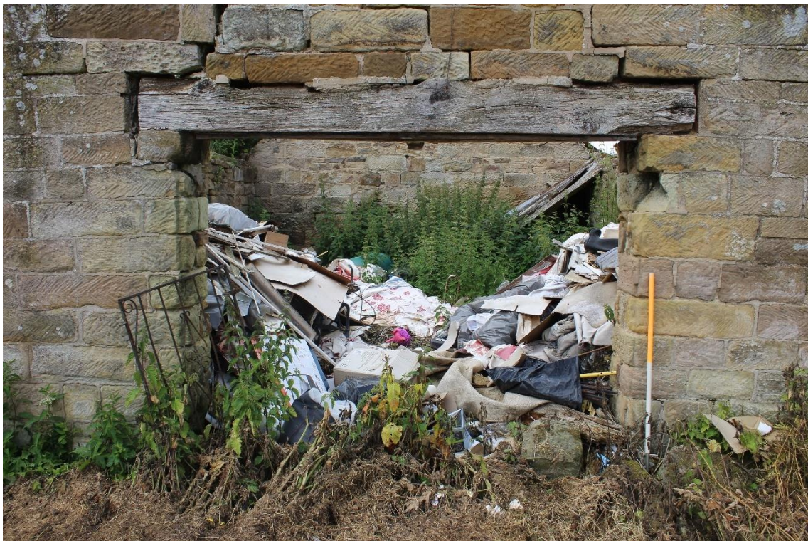
Plate 100: Exterior close up view E elevations of Building No. 2 and internal area
