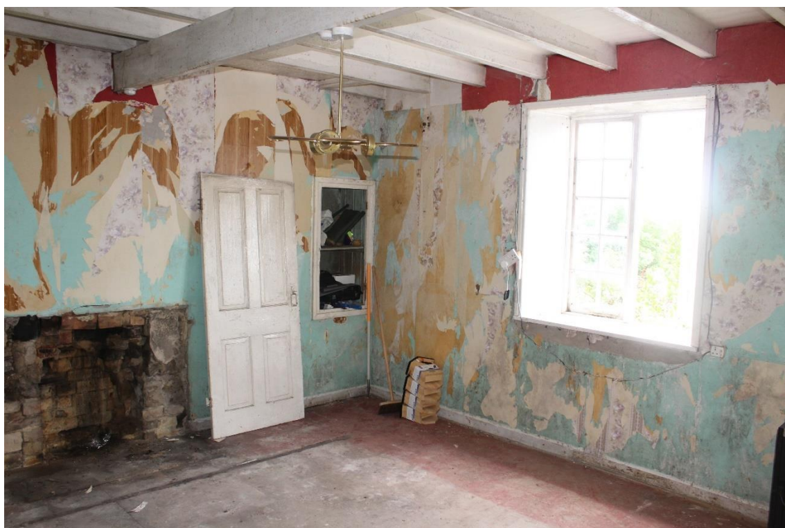
Plate 38: internal view SE within ground sitting room – Building No. 1
