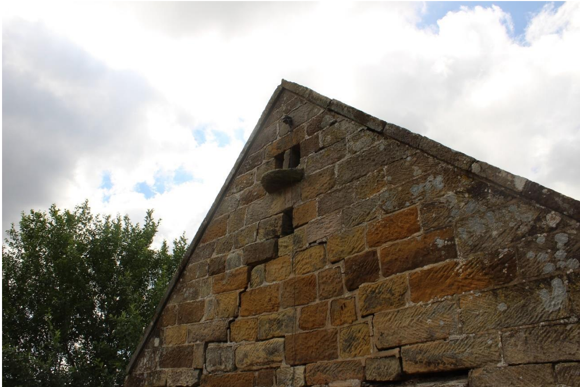
Plate 101: Exterior close up view showing nesting holes within E elevations of Building No. 2
