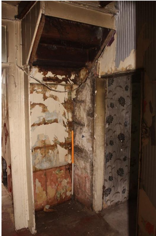
Plate 17: Internal view S within the ground floor of the central halls N compartment – Building No. 1
