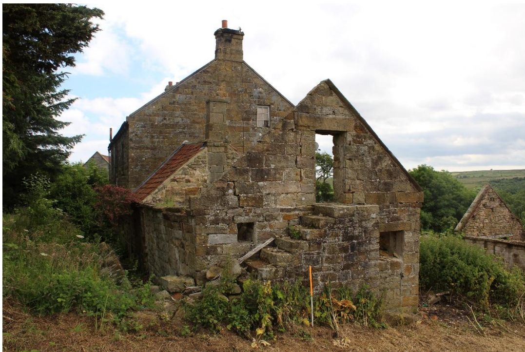
Plate 7: View E showing W facing and N facing elevations of Building No. 1. Pigsty and out building in foreground, main farmhouse in background
