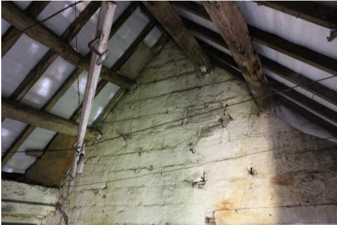
Plate 51: internal view NW within ground floor outhouse showing ceiling
