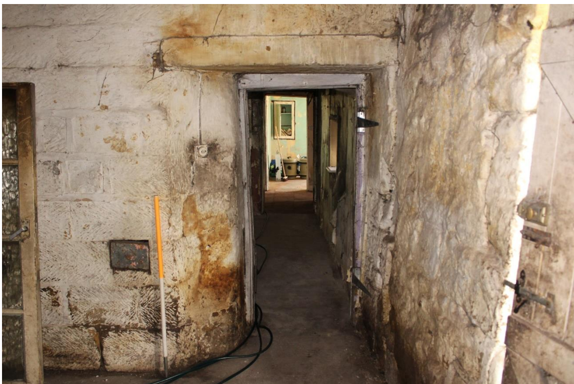
Plate 50: internal view NW within ground floor outhouse showing entrance from kitchen and soot box – Building No. 1
