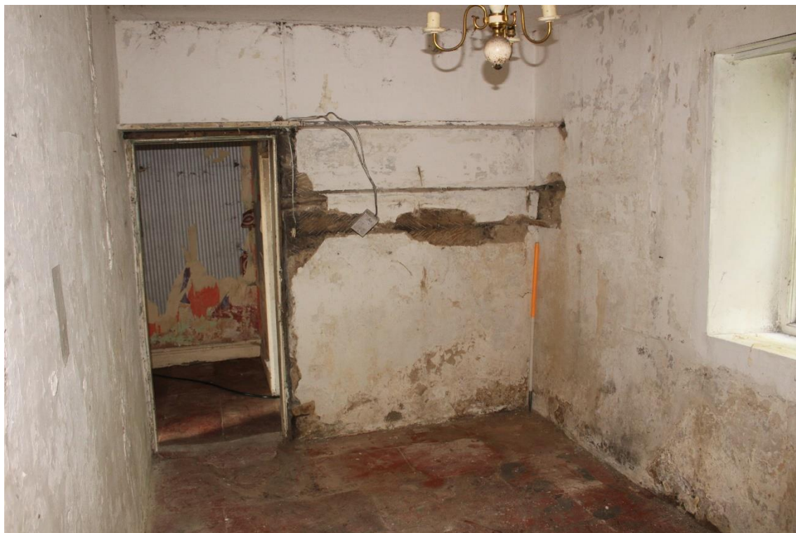
Plate 35: internal view WSW within ground floor storage room— Building No. 1
