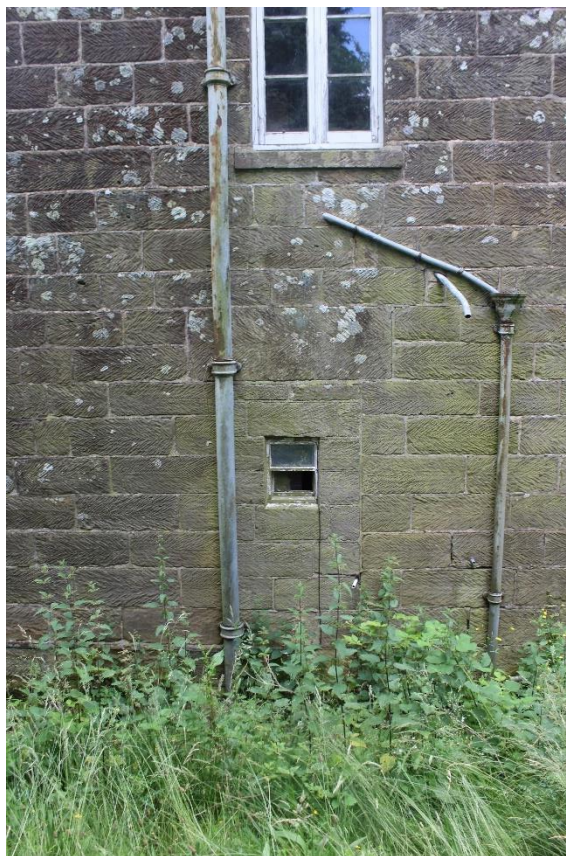
Plate 10: View SSE showing blocked central door within N facing elevation of the farmhouse (Building No. 1)
