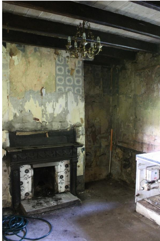
Plate 25: internal view WNW within ground floor kitchen – Building No. 1
