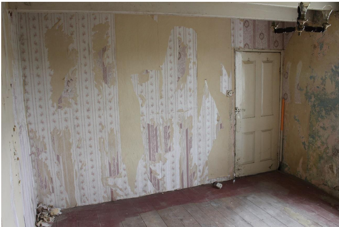
Plate 66: Internal view ESE of 1 st floor bedroom– Building No.1
