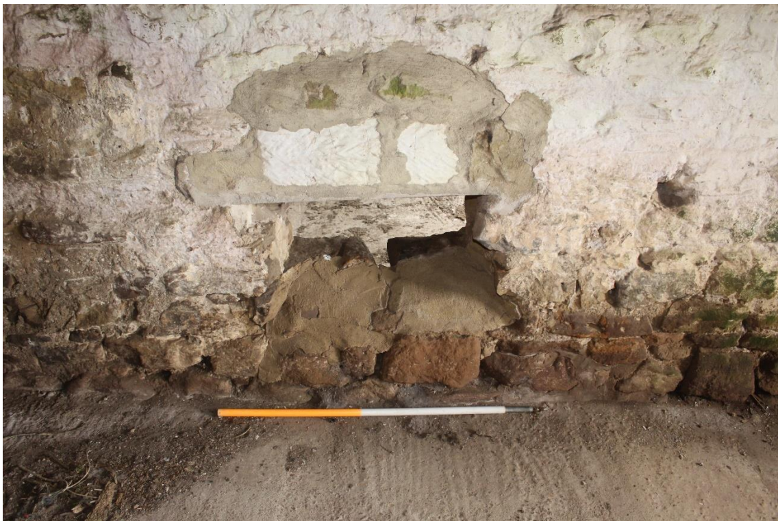
Plate 134: Internal view E of hole in E wall within the first compartment of Building No.4
