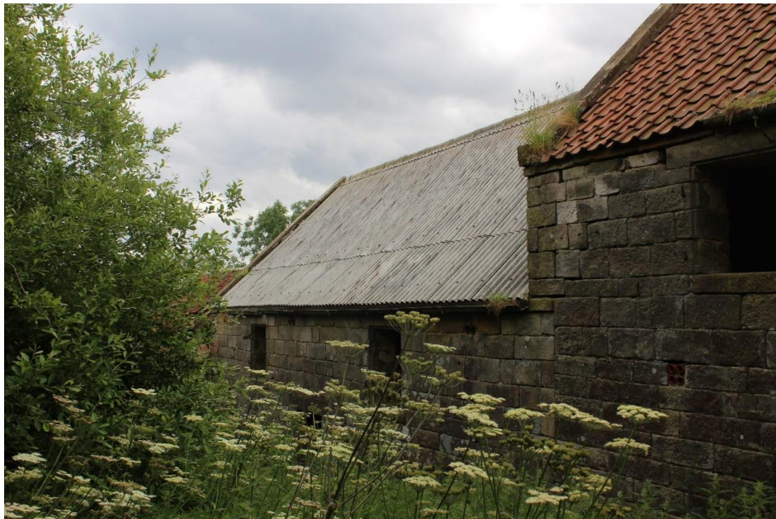
Plate 125: Oblique external view SSE of N-facing elevation of Building No.4
