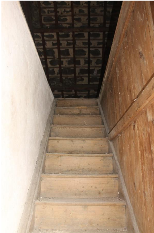
Plate 87: Internal view NNW of stair case leading to attic/roof space – Building No.1
