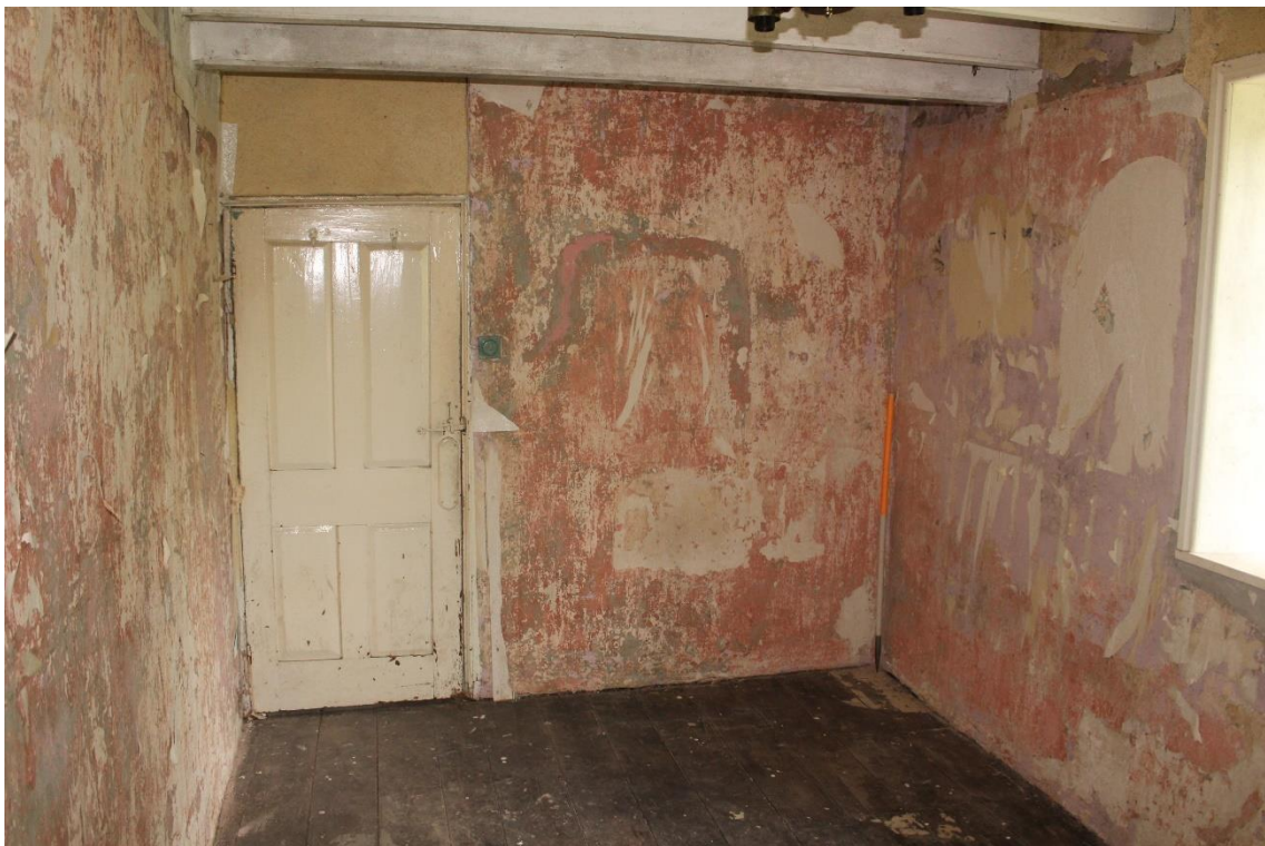
Plate 78: Internal view WSW of 1st floor third bedroom – Building No.1
